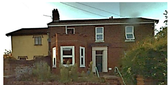
View of the elevation of 145
