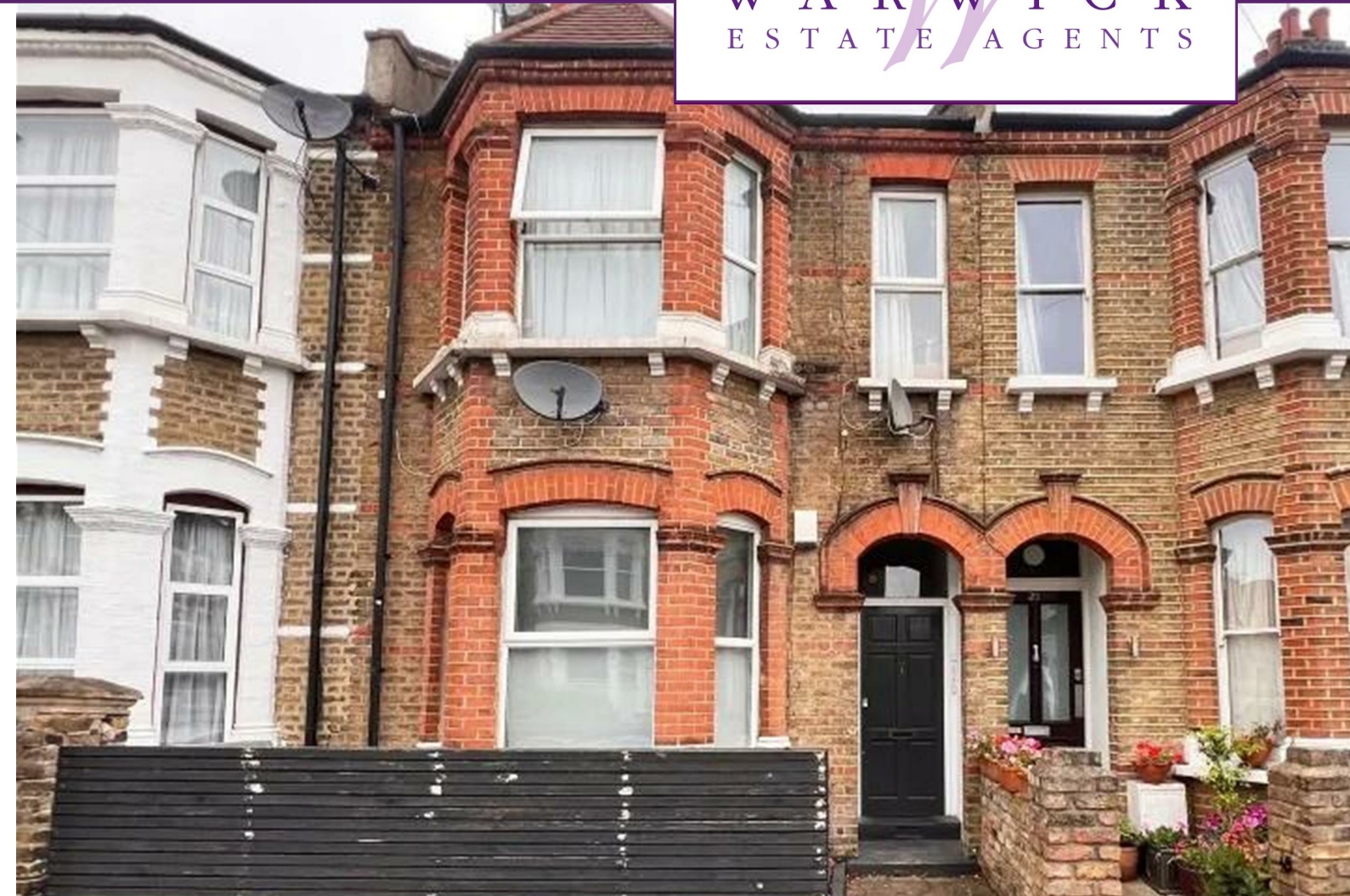
Ashburnham Road, London, NW10 5SB
