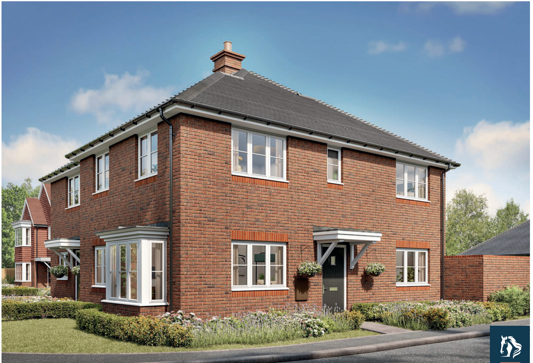
The Grange ~ Plot 9 attached to Plot 10
