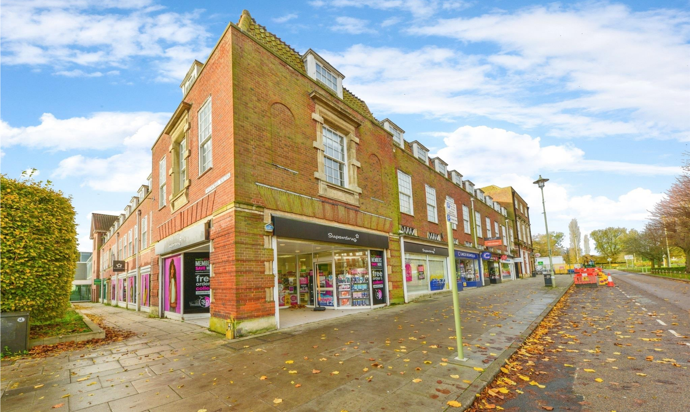
Windsor House Howardsgate, Welwyn Garden City AL8 6DJ
