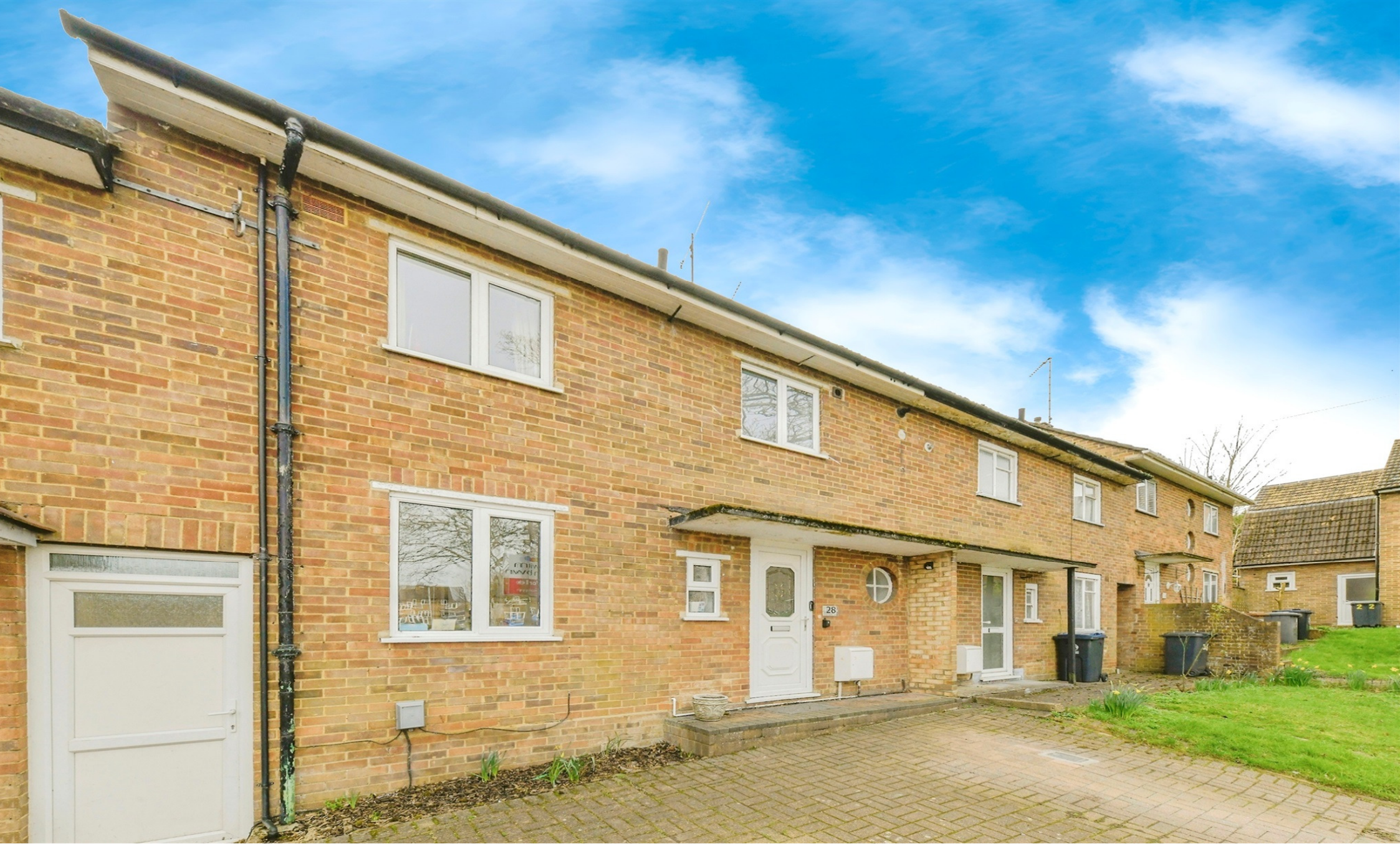
Red House Close, Ware SG12 9NW
