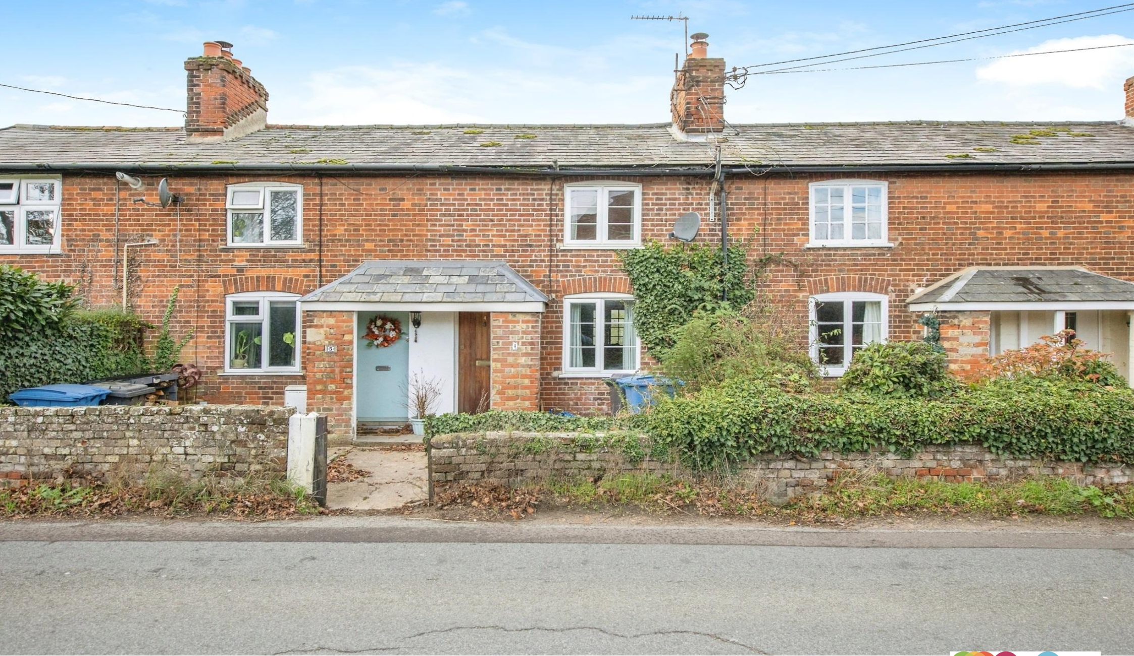
Chilton Corner Cottages, Valley Road, Great Waldingfield, Sudbury CO10 0RH
