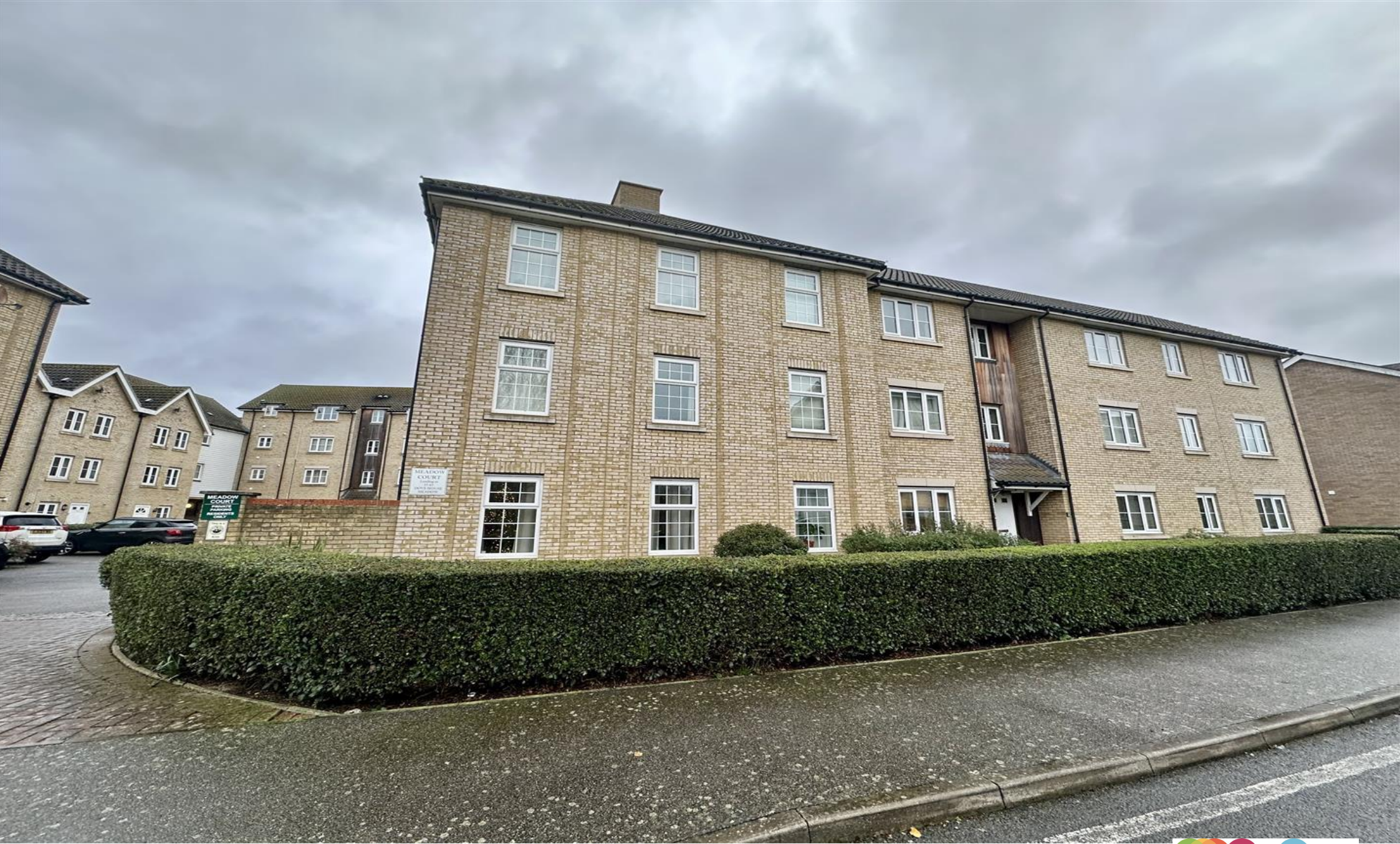
Dove House Meadow, Great Cornard, Sudbury CO10 0GF
