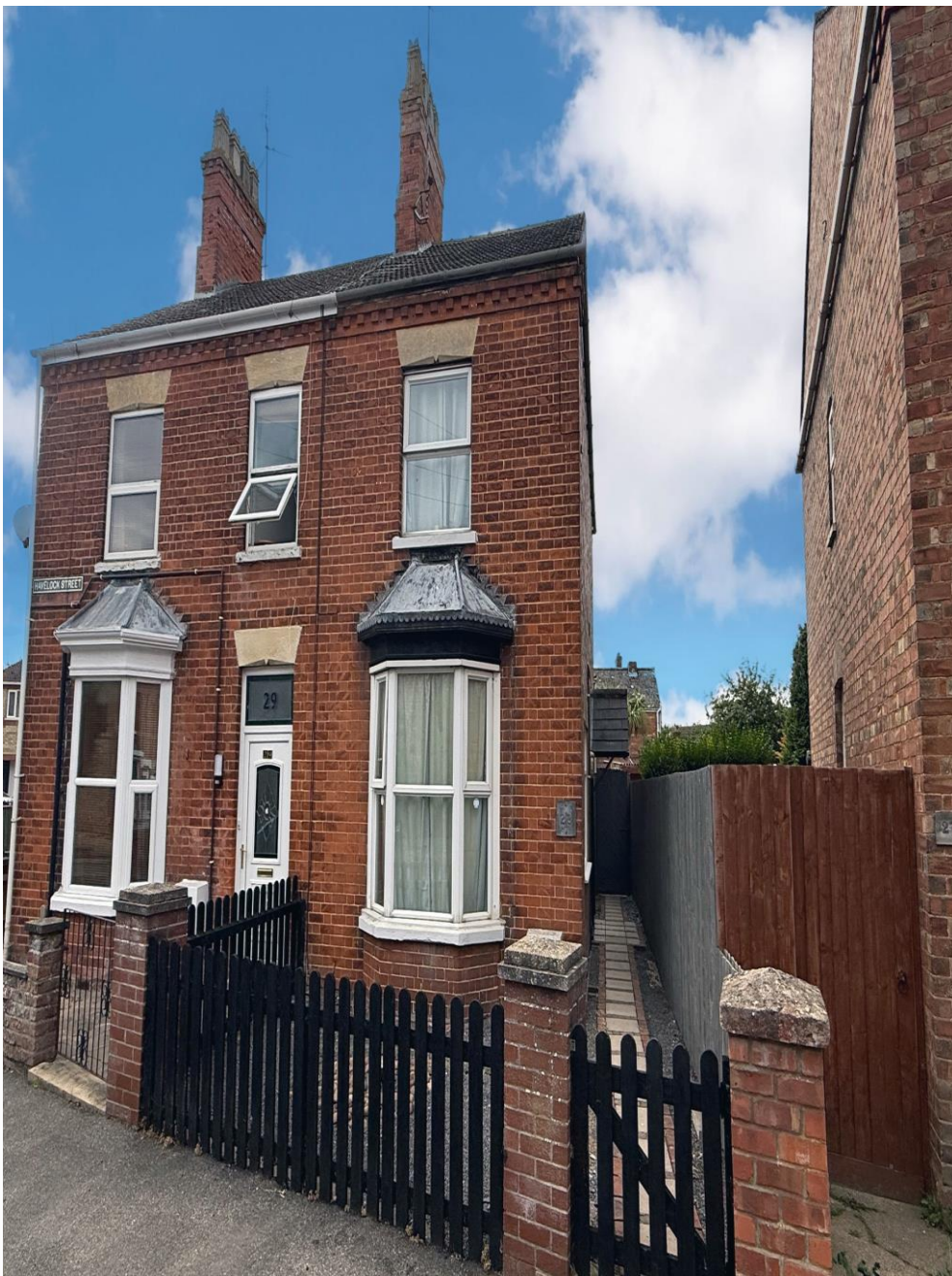
Havelock Street, Spalding PE11 2YL
