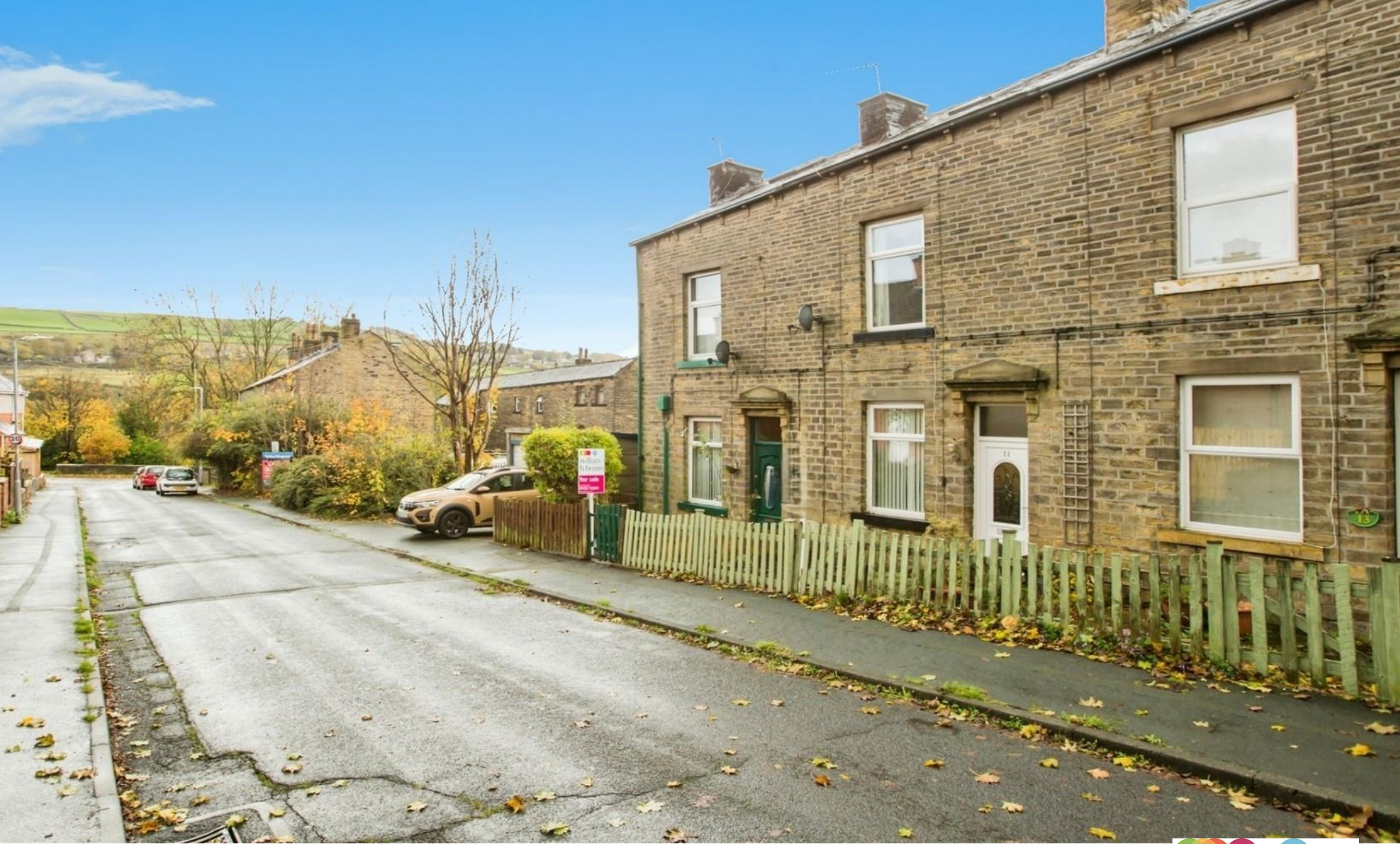
Belmont Street, Sowerby Bridge, HX6 2DB
