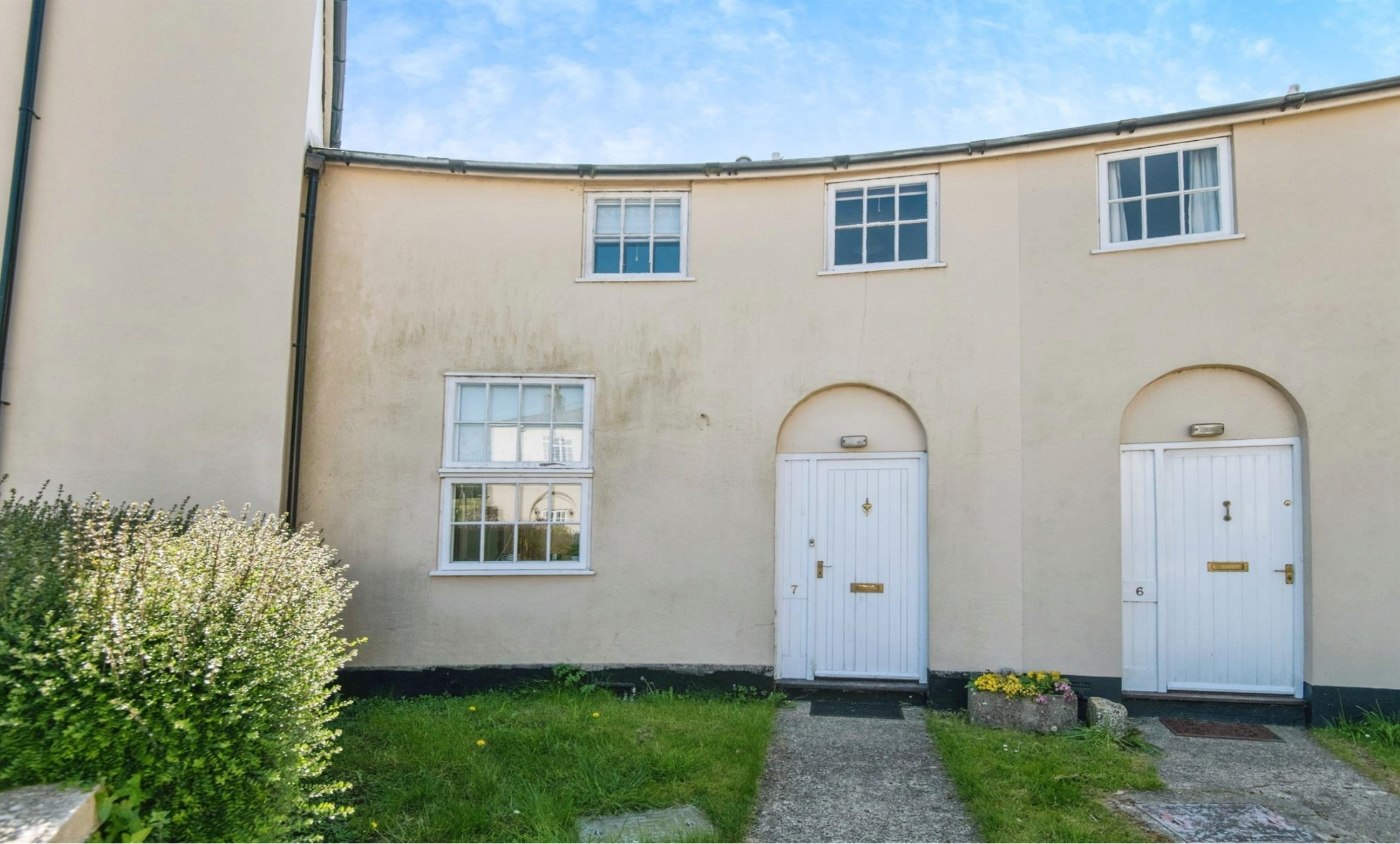
The Stables Shute, Axminster EX13 7NY
