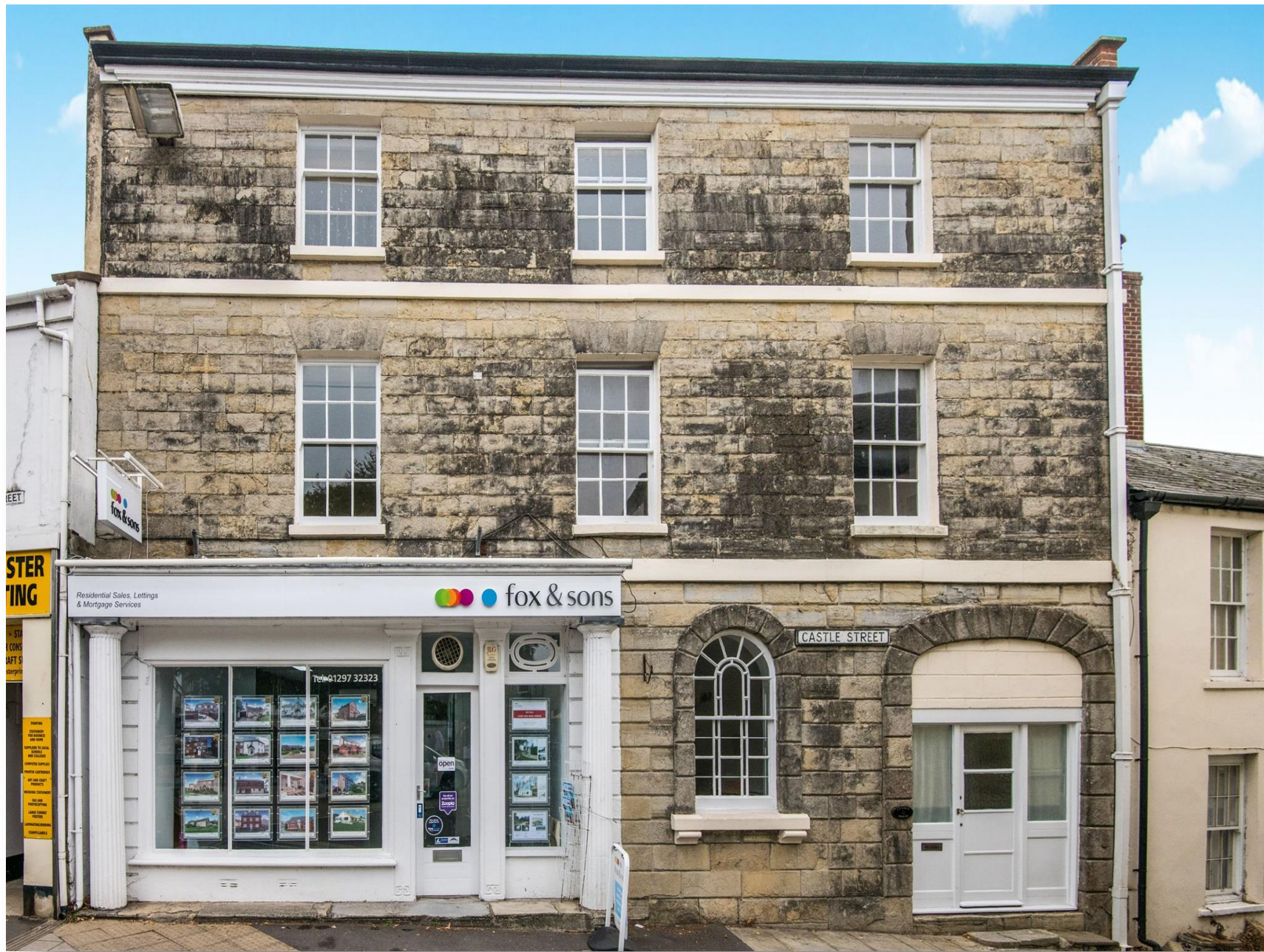
Estate House West Street, Axminster EX13 5NU
