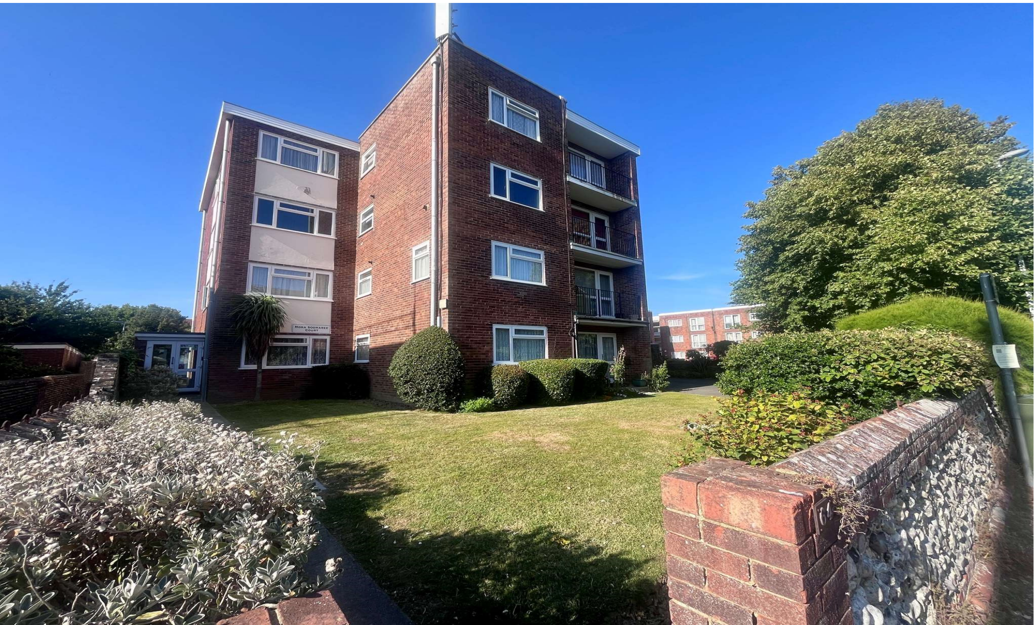
Mora Soomaree Court Shelley Road, Worthing BN11 4DF
