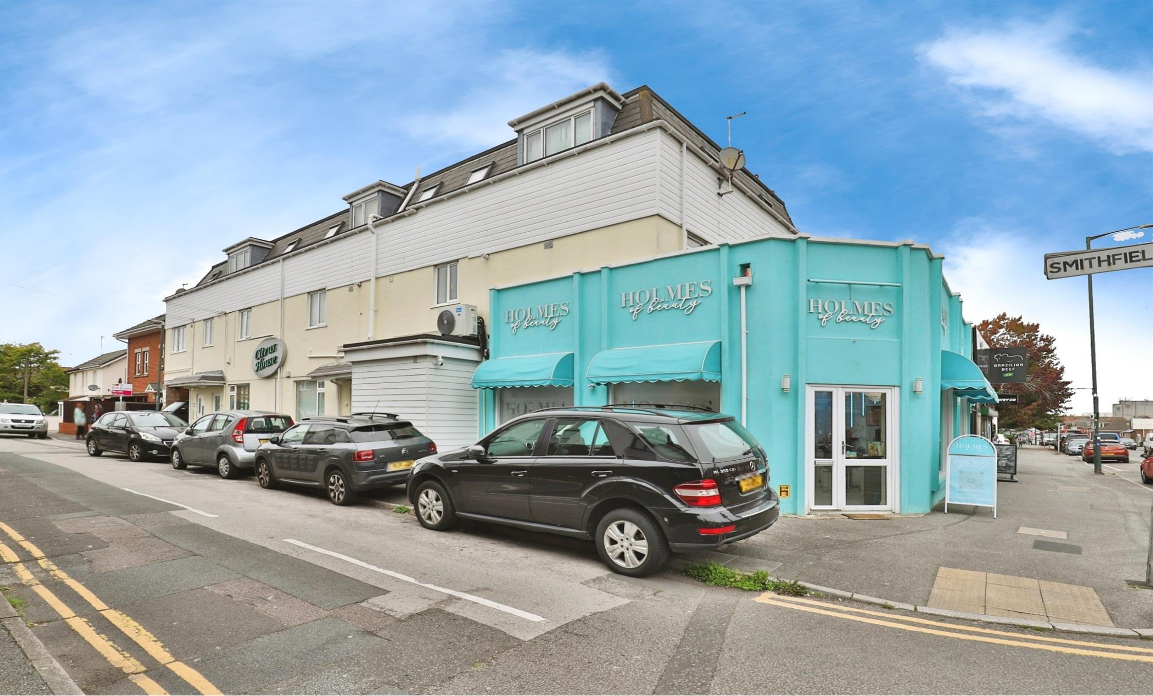
Citrus House Wimborne Road, Bournemouth BH9 2EN
