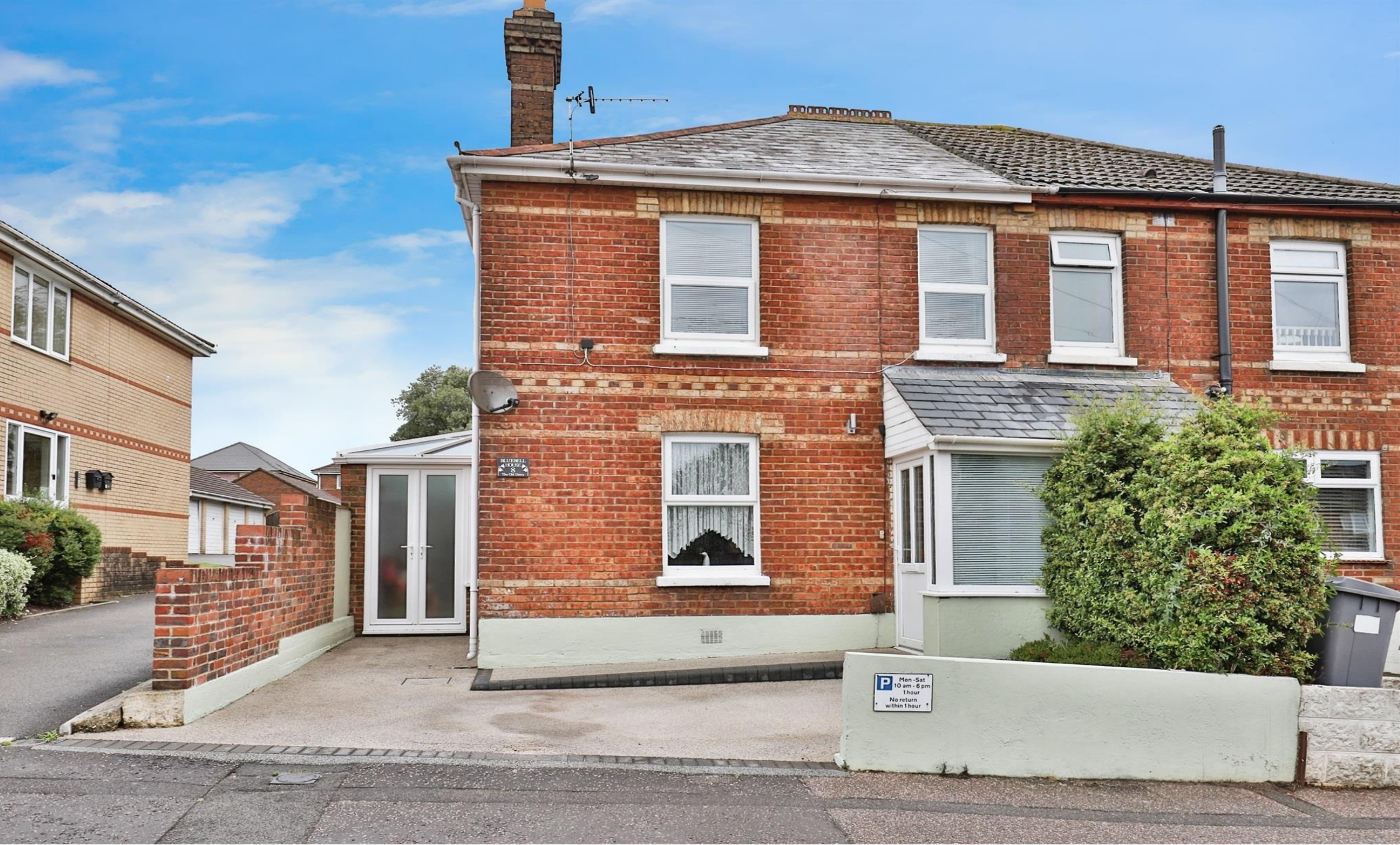
Luther Road, Bournemouth BH9 1LH
