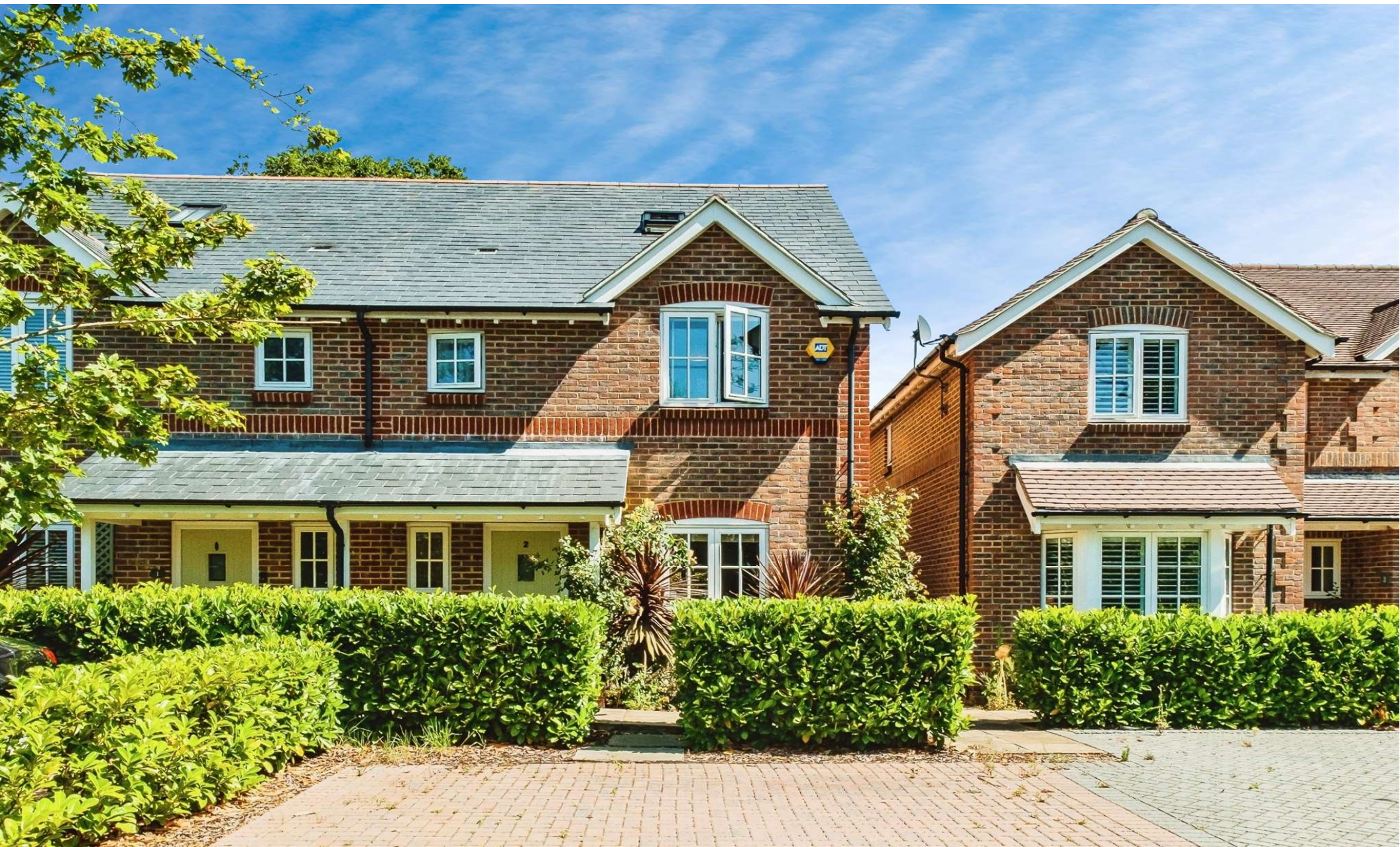
Brickyard Cottages Long Furlong, Clapham Worthing BN13 3XU
