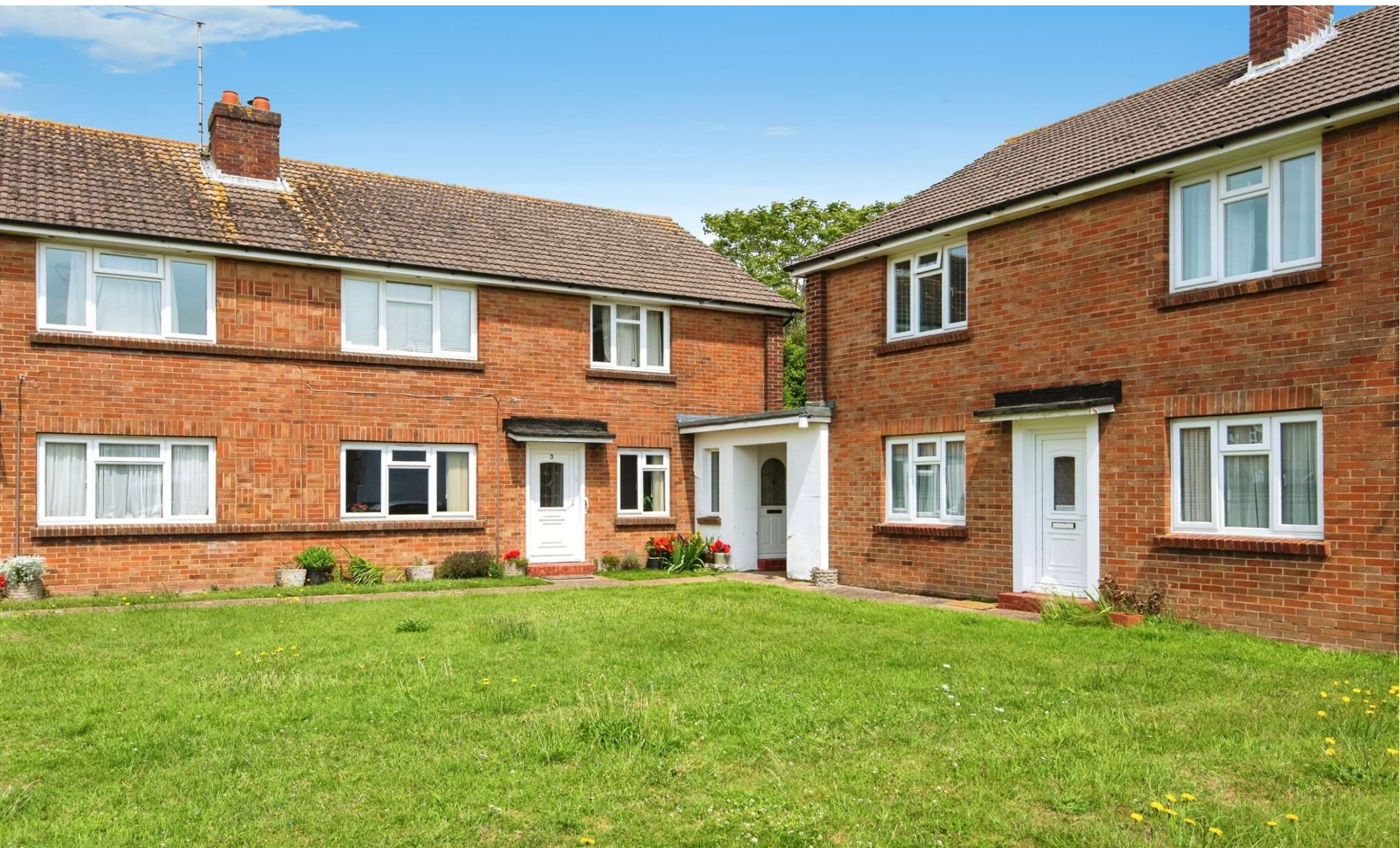
Dolphin Court Canterbury Road, Worthing BN13 1AF
