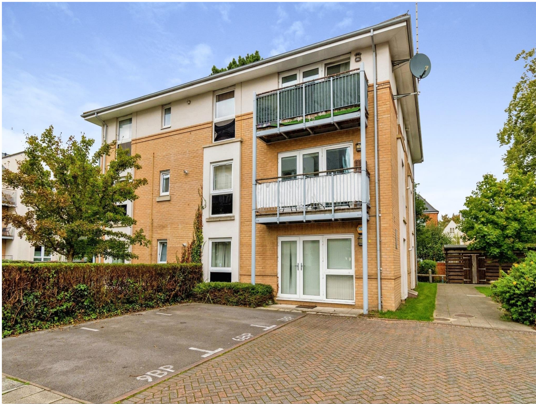
Bourne Place, Archers Road, Southampton SO15 2LR
