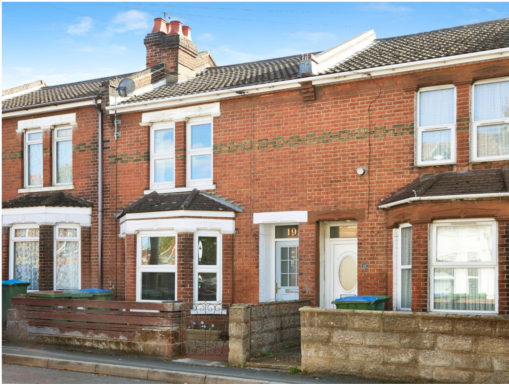
Foundry Lane, SOUTHAMPTON SO15 3FX
