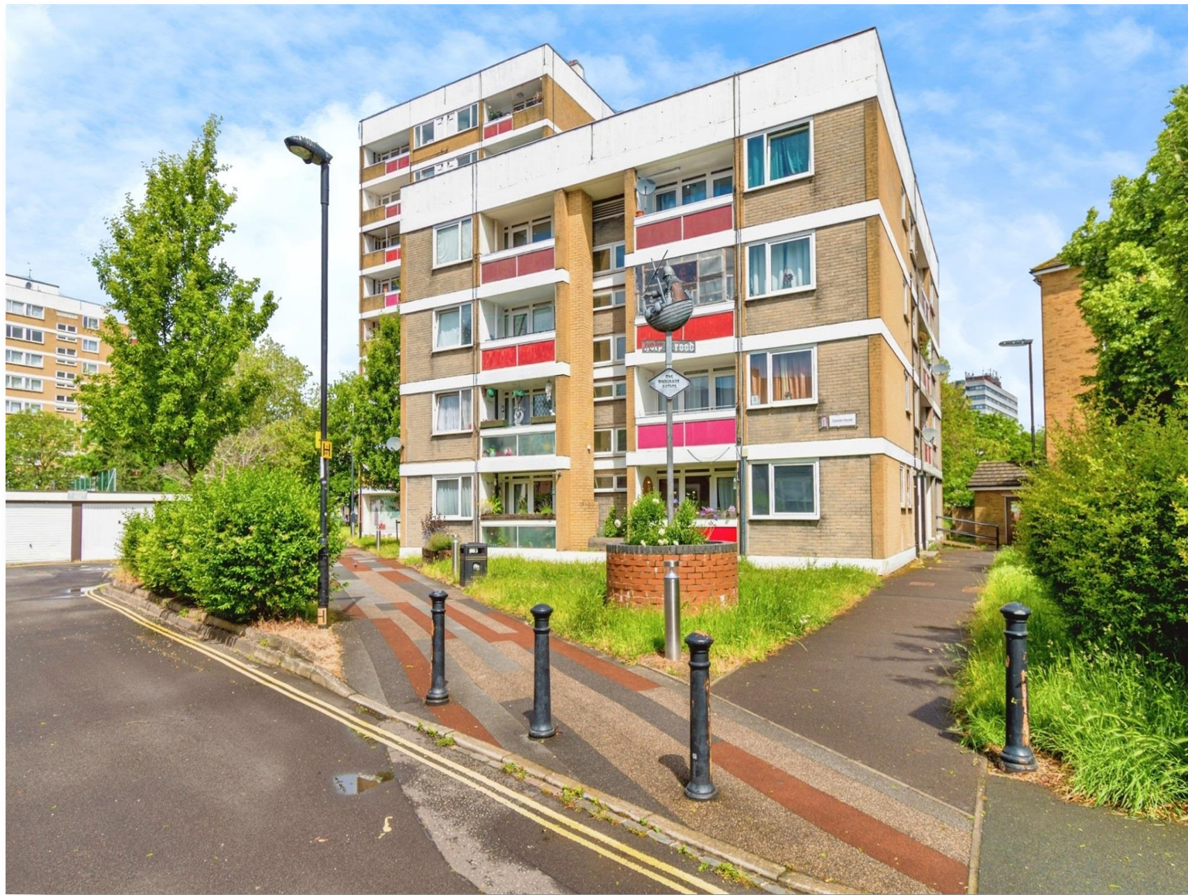
Canute House King Street, Southampton SO14 3DG
