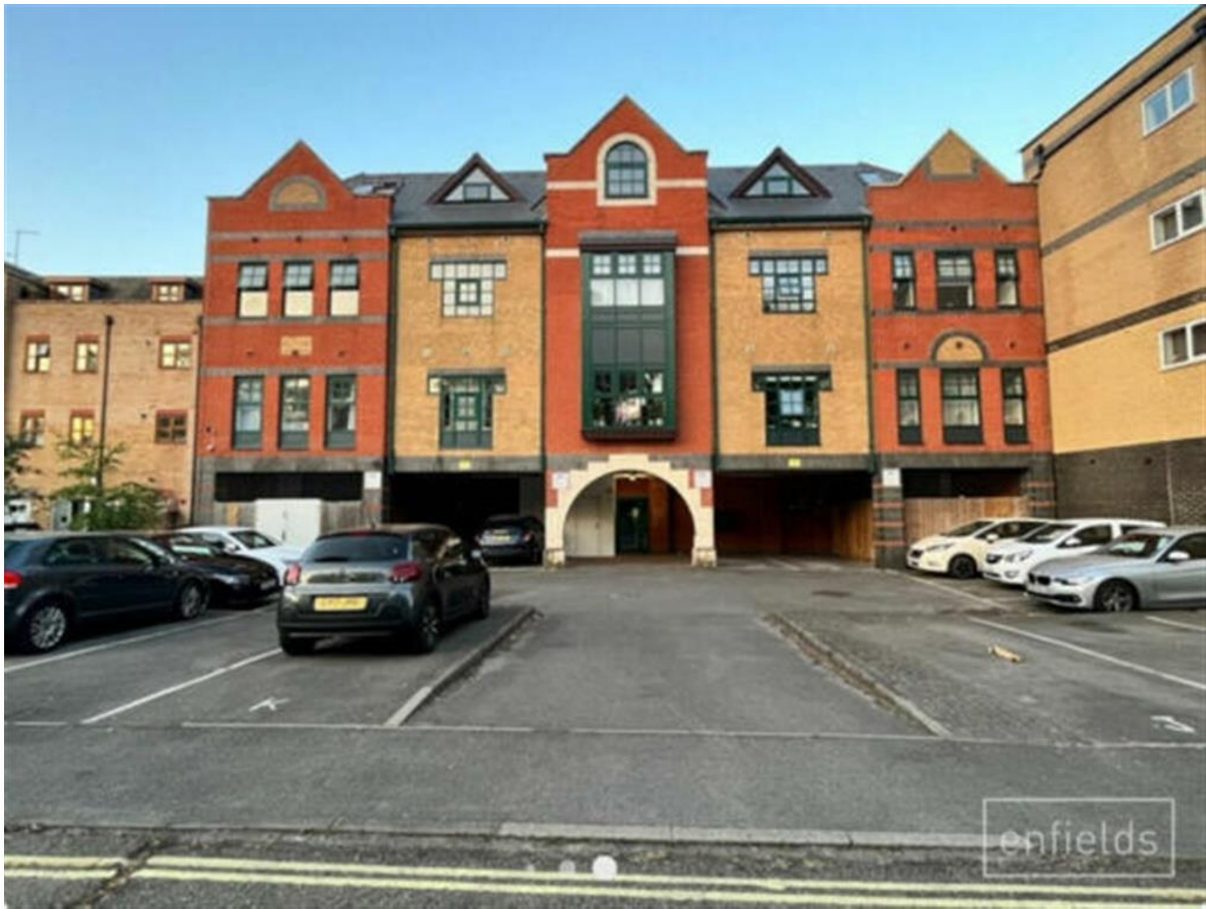
Hampton House St. Marys Place, Southampton SO14 1AZ
