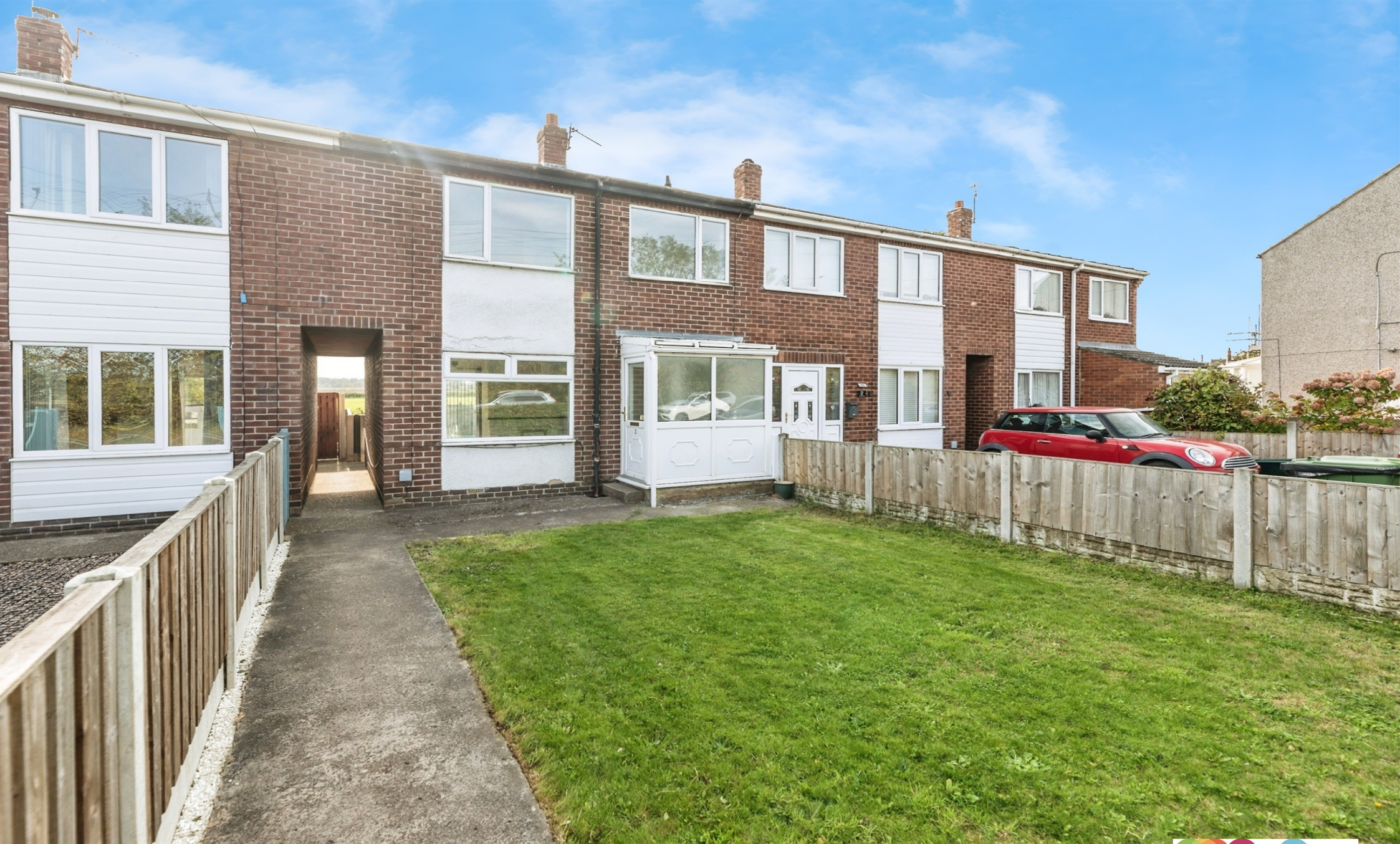
Snydale Villas, Streethouse Pontefract WF7 6BU
