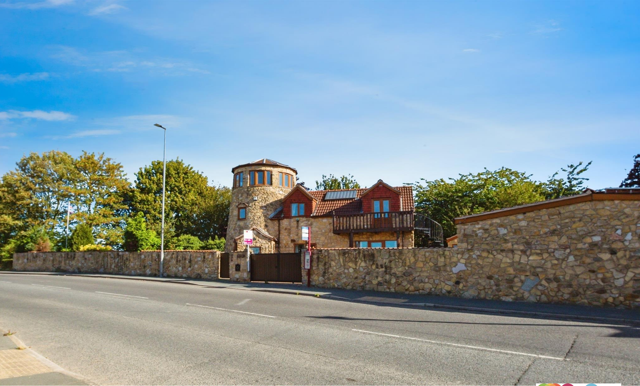
The Mill Mill Lane, South Elmsall Pontefract WF9 2DU
