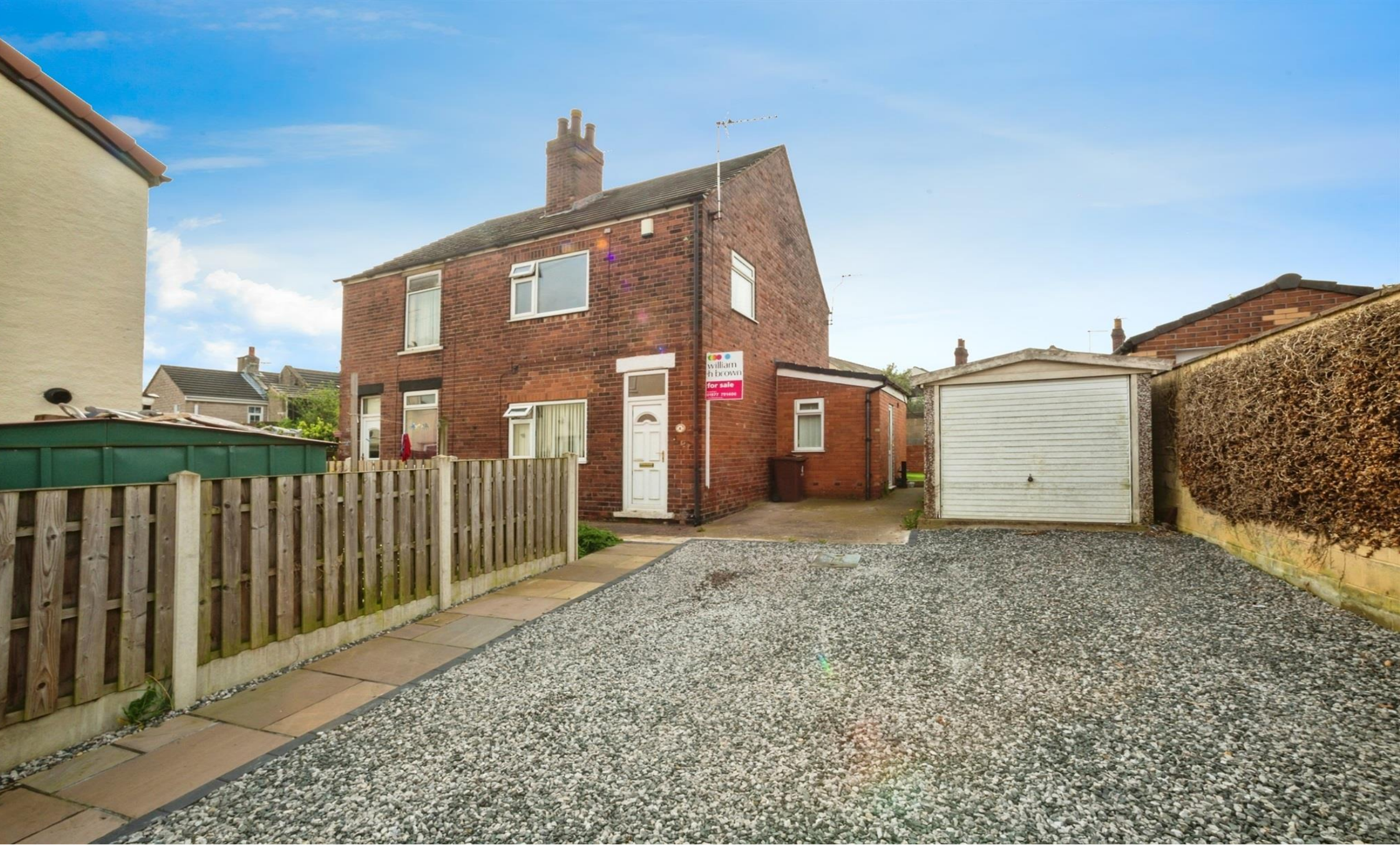
Chapel Yard, Knottingley WF11 8HW
