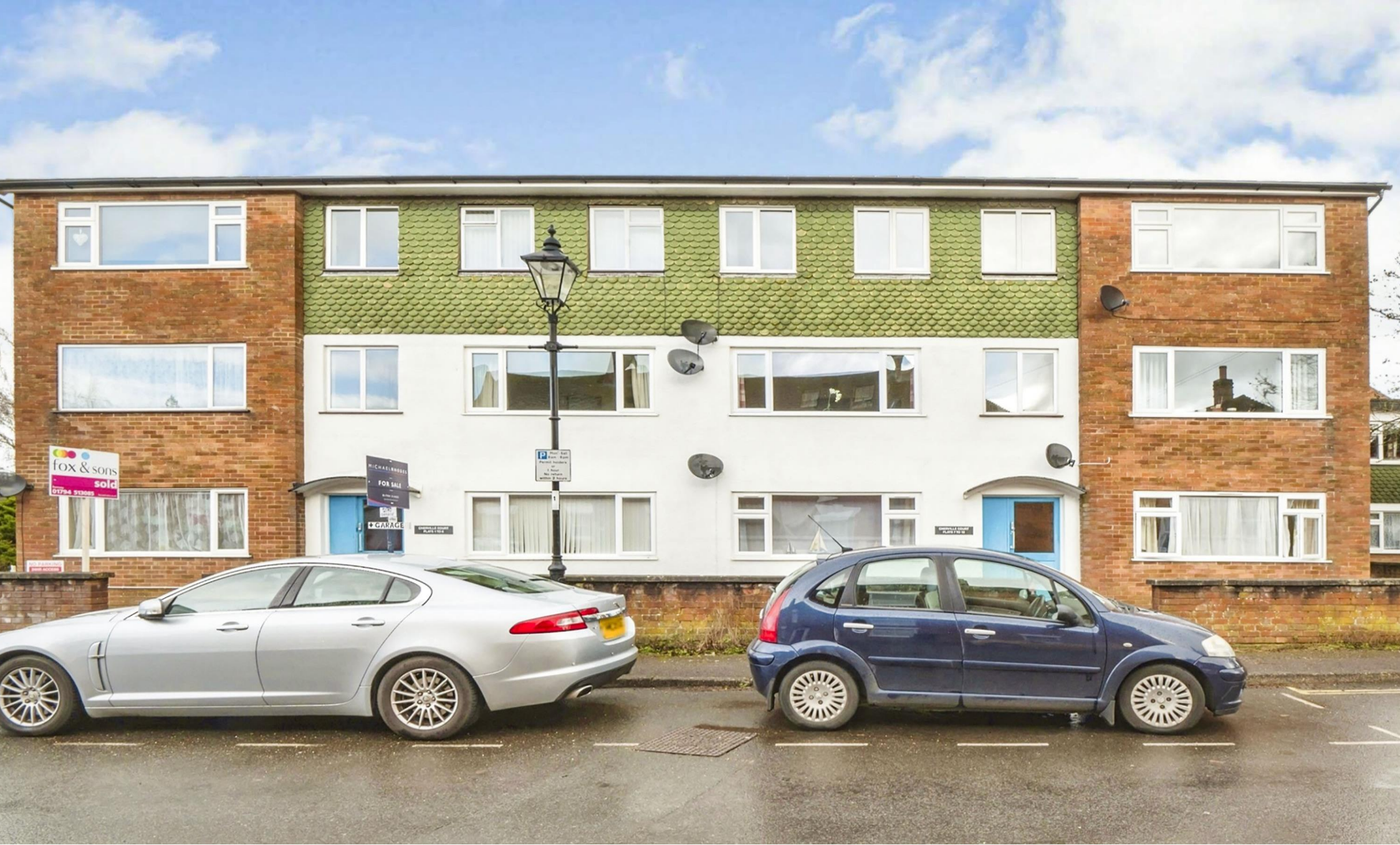
Cherville Court, Mill Lane, Romsey, SO51 8EX
