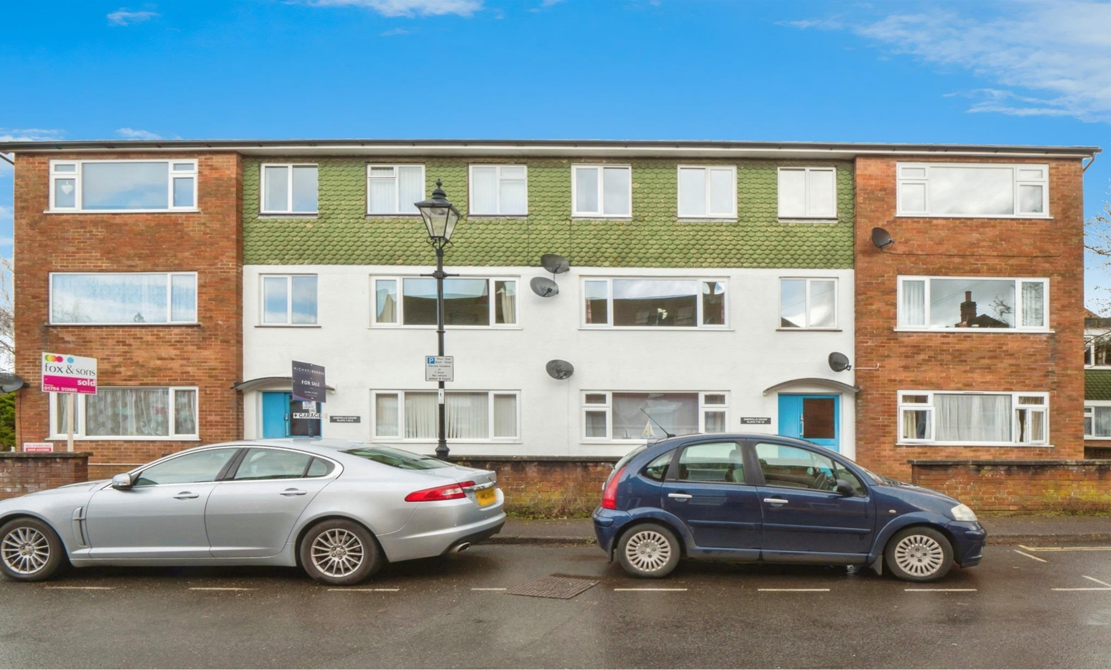
Cherville Court, Mill Lane, Romsey, SO51 8EX
