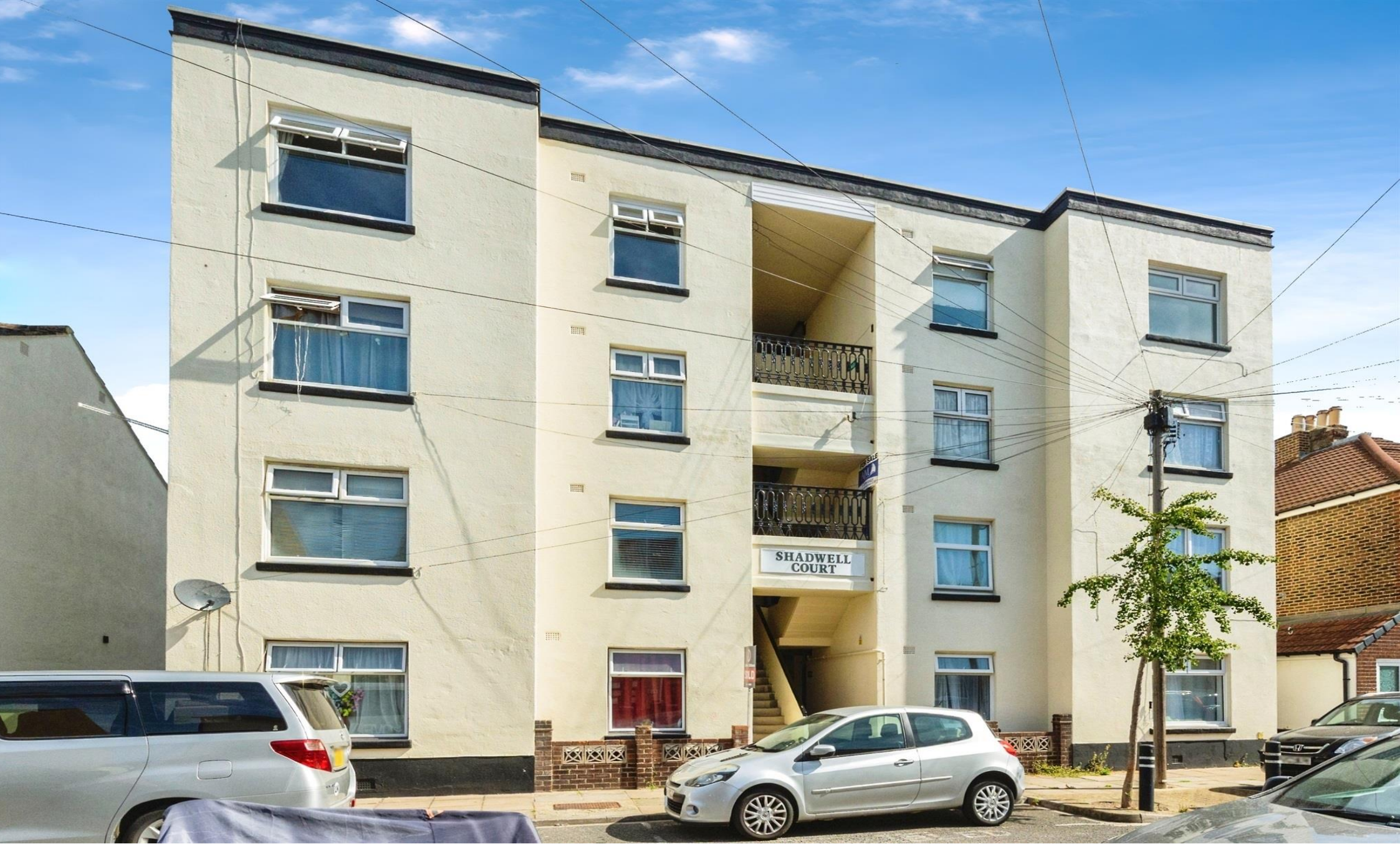
Shadwell Court Winstanley Road, Portsmouth PO2 8JU
