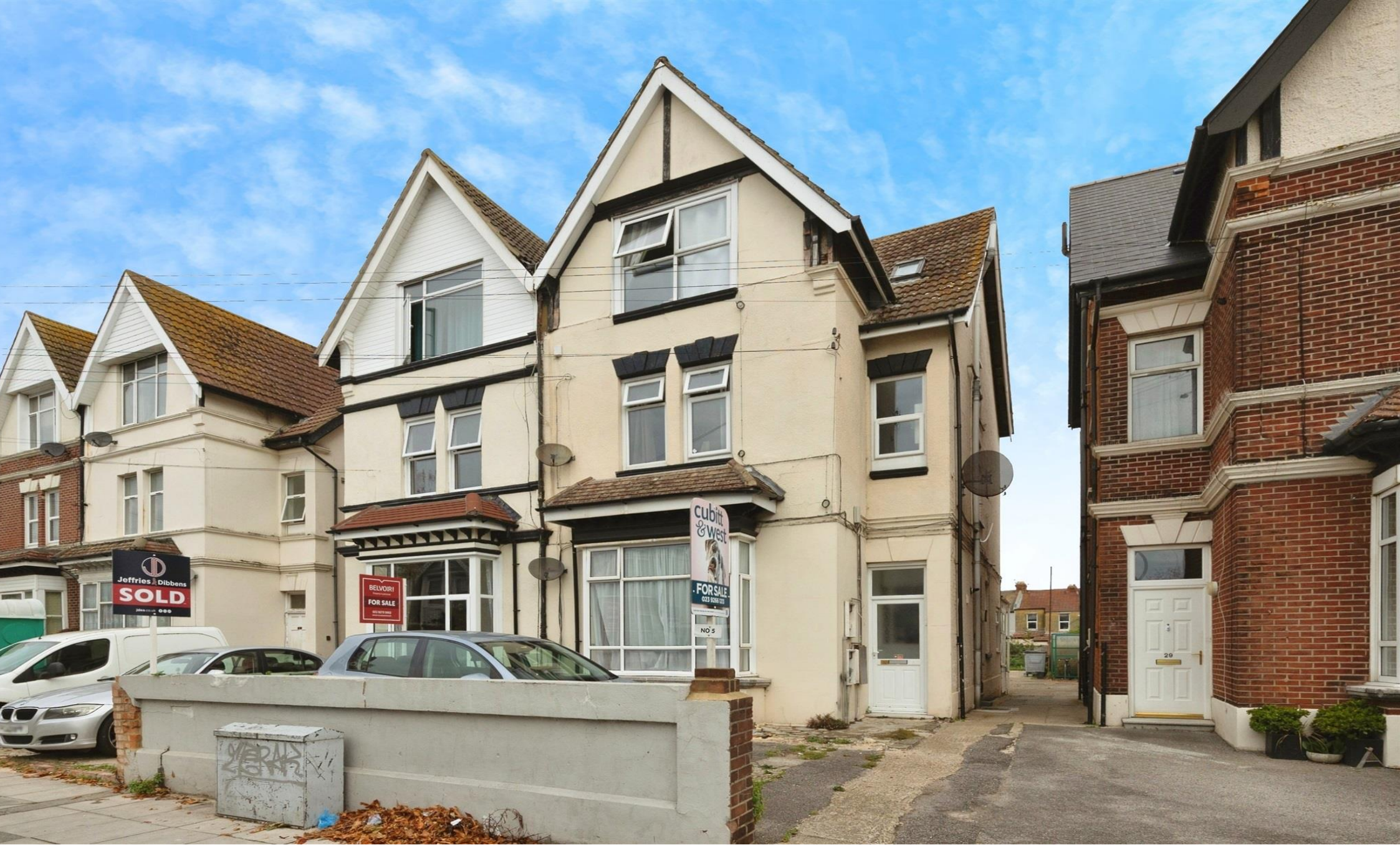
Stubbington Avenue, Portsmouth PO2 0HP
