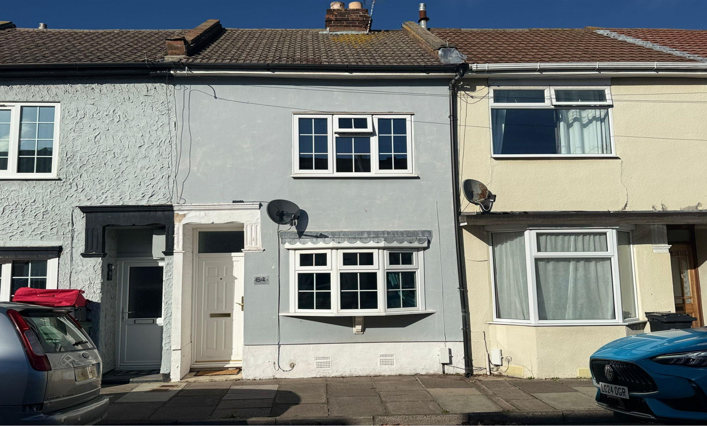
Ranelagh Road, PORTSMOUTH PO2 8HA
