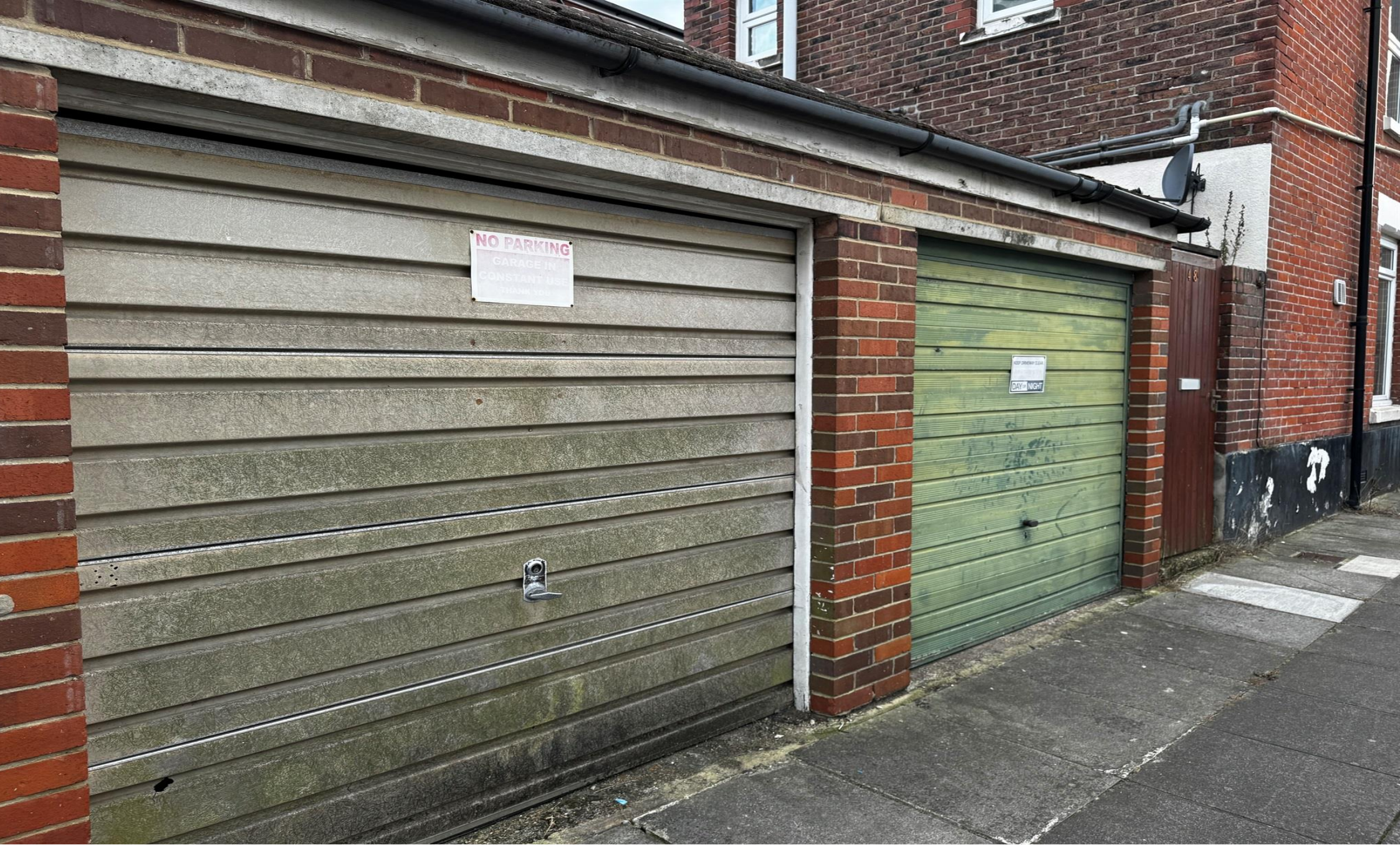
The Garages Whitworth Road, Portsmouth PO2 7RU
