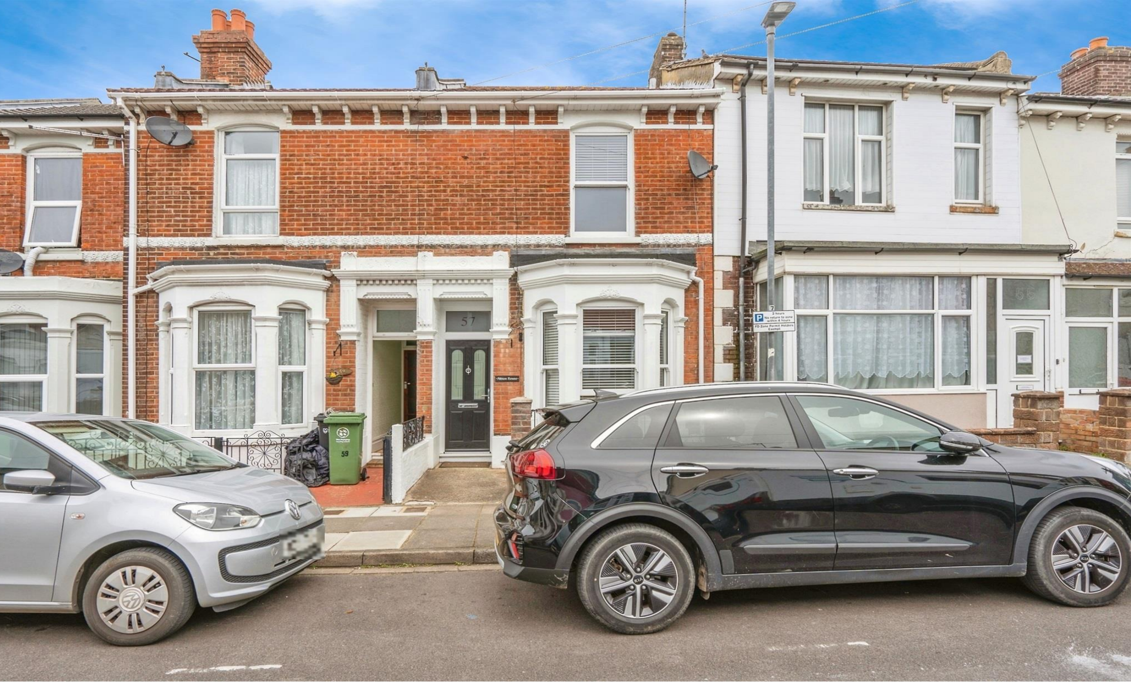
Pitcroft Road, Portsmouth PO2 8BB
