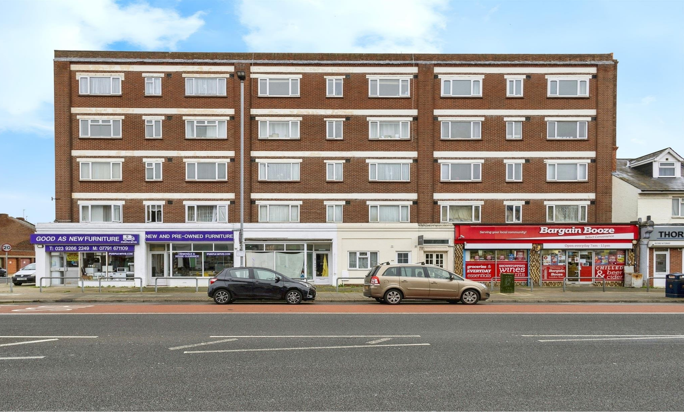
Vernon Court London Road, Portsmouth PO2 9JR
