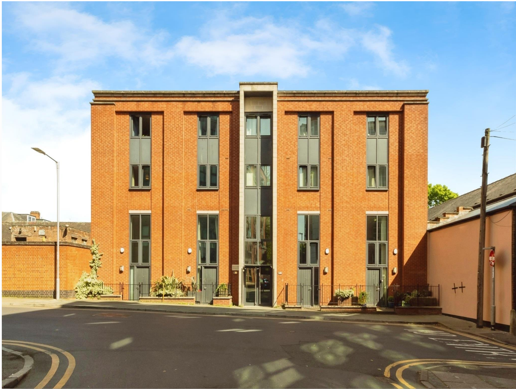
Hockley House Woolpack Lane, Nottingham NG1 1GA
