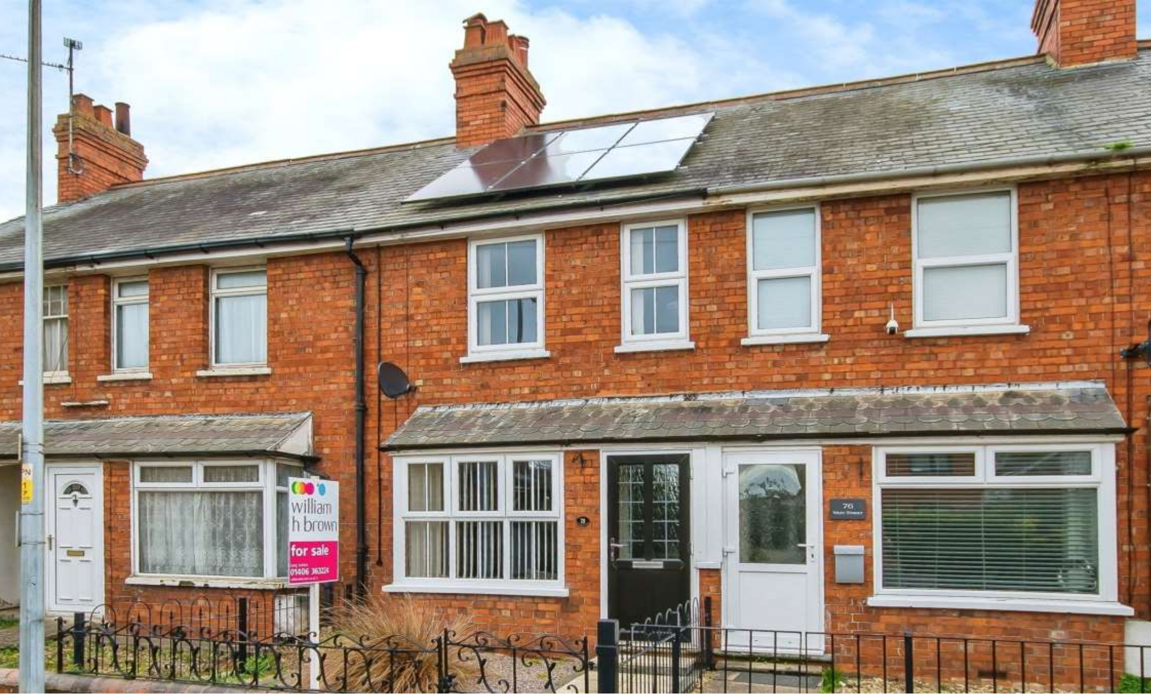
West Street, Long Sutton Spalding PE12 9BN
