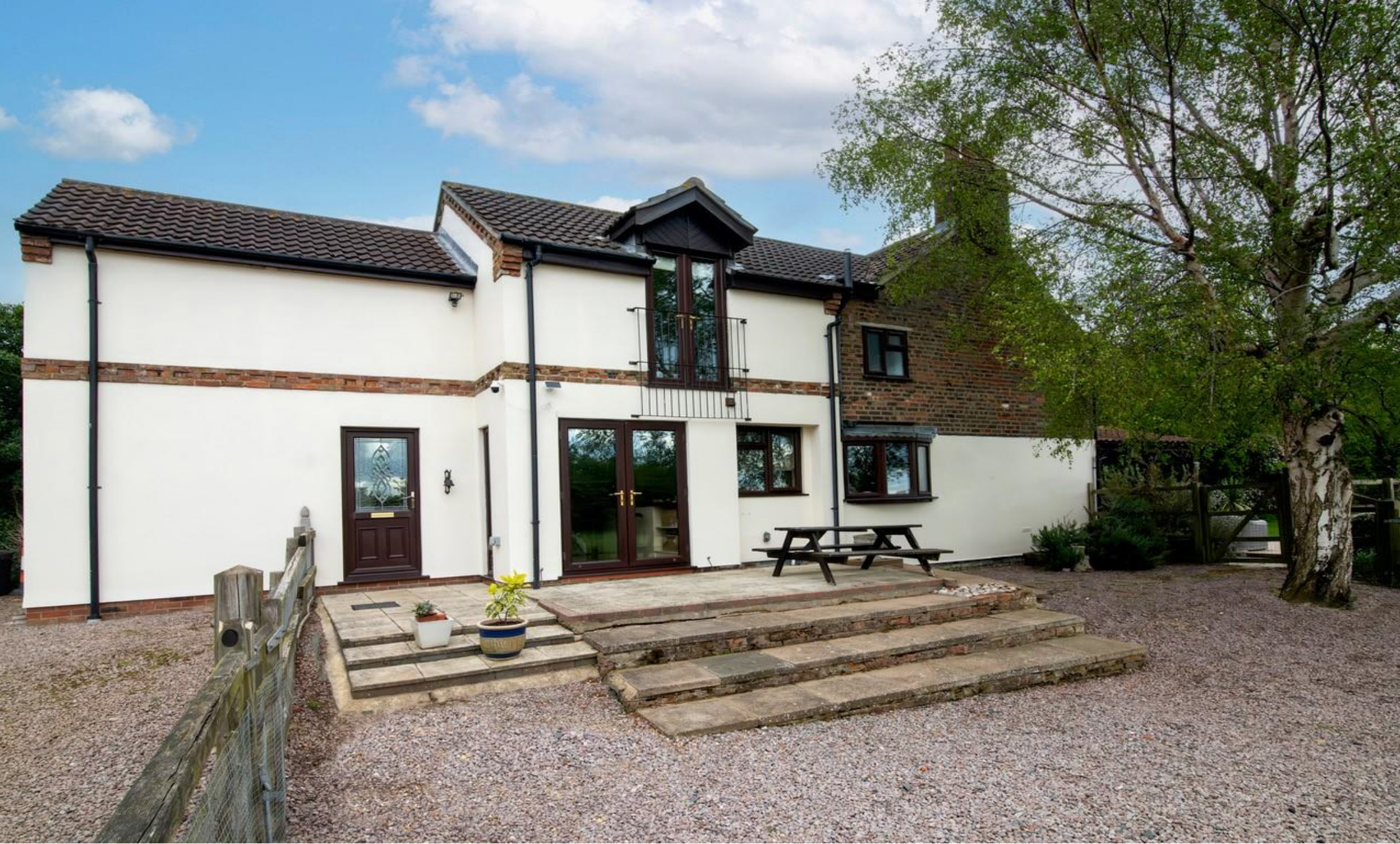
Old Cottage Lutton Bank, Lutton Spalding PE12 9LJ
