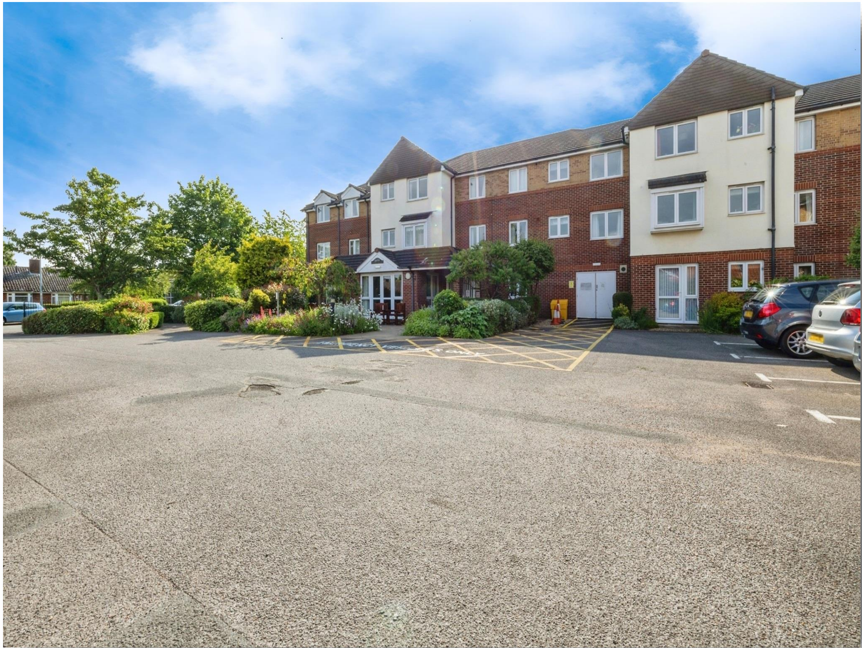
Cathedral View Court, Lincoln LN2 2GF
