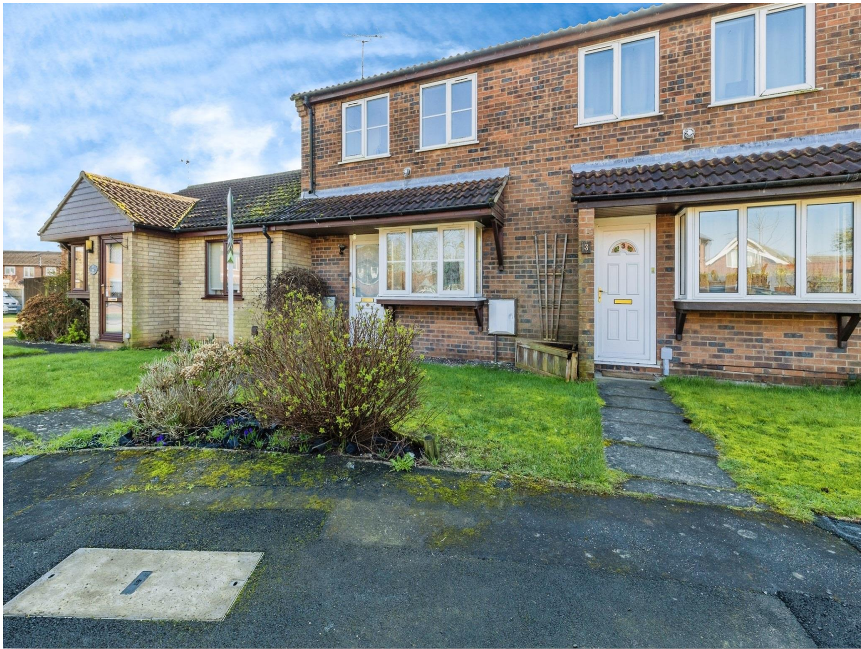
Bramble Court, Bracebridge Heath Lincoln LN4 2QY
