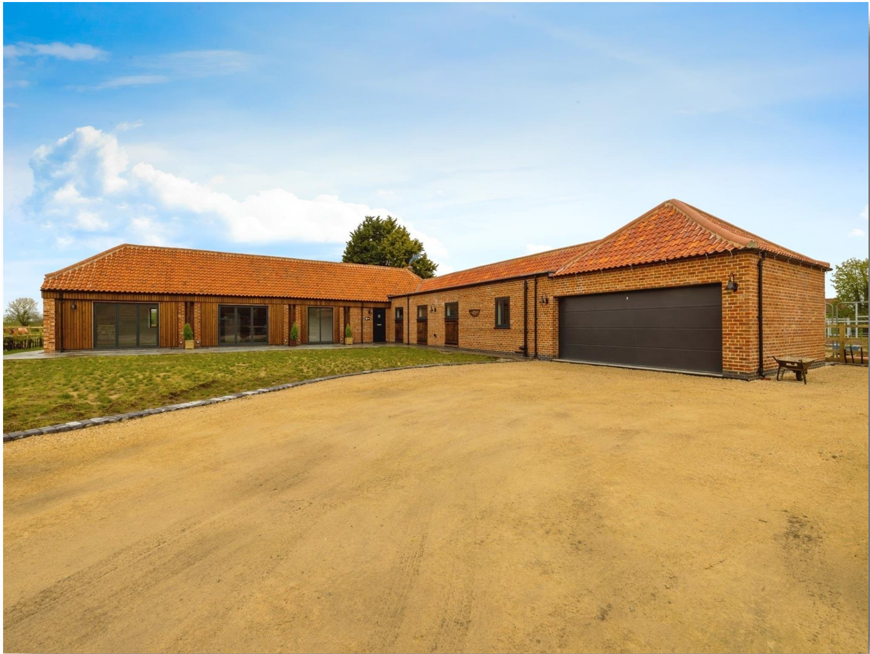
Manor Farm Yard Main Street, Timberland Lincoln LN4 3RZ
