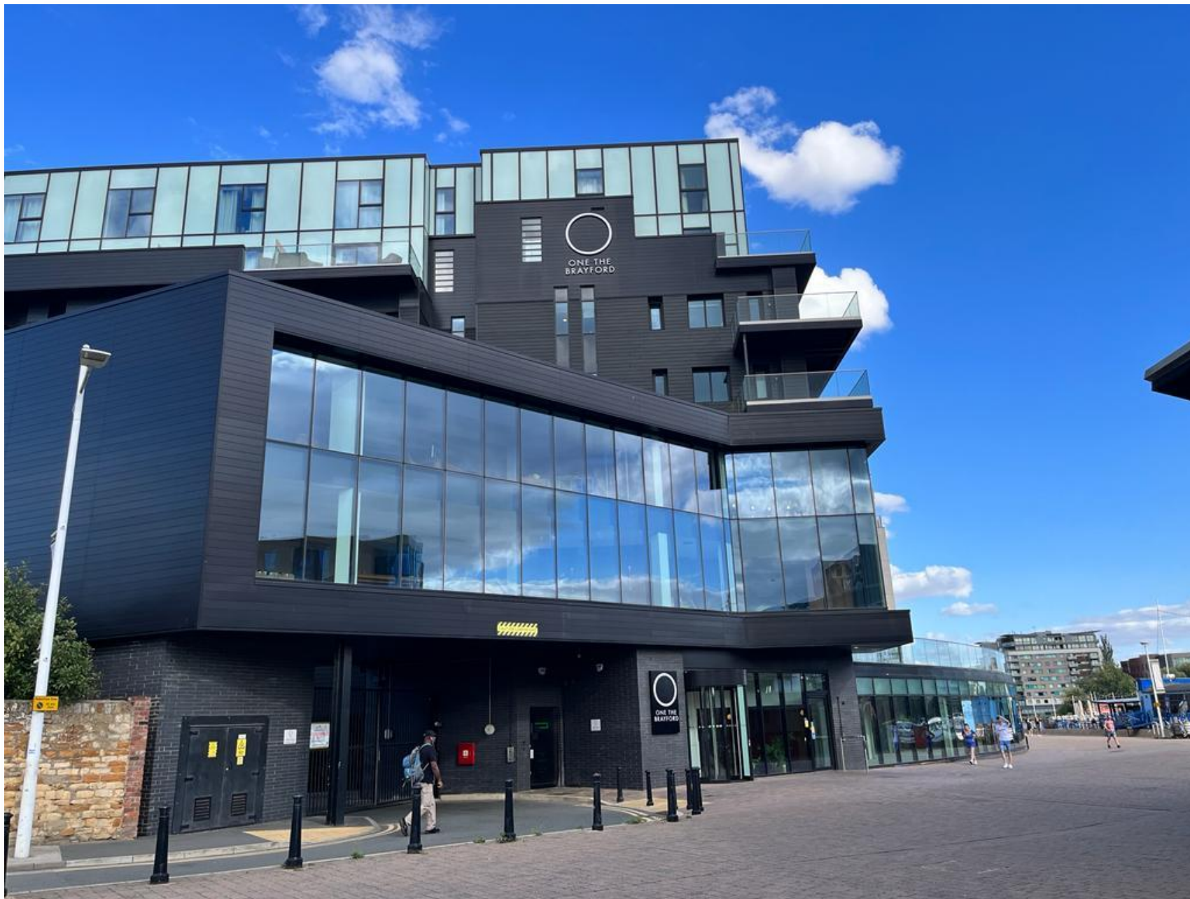
One The Brayford Brayford Wharf North, Lincoln LN1 1BN
