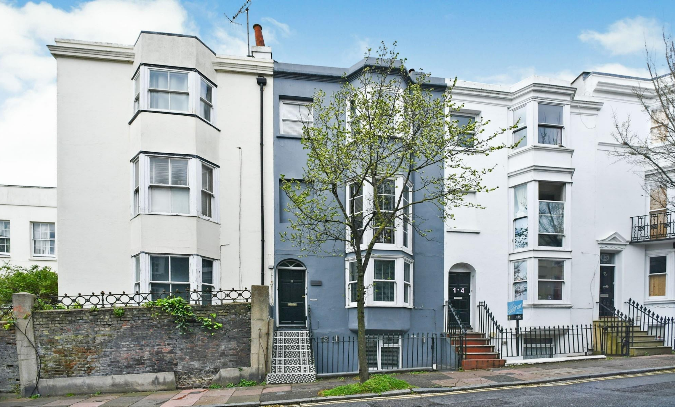
Basement Egremont Place, Brighton BN2 0GA
