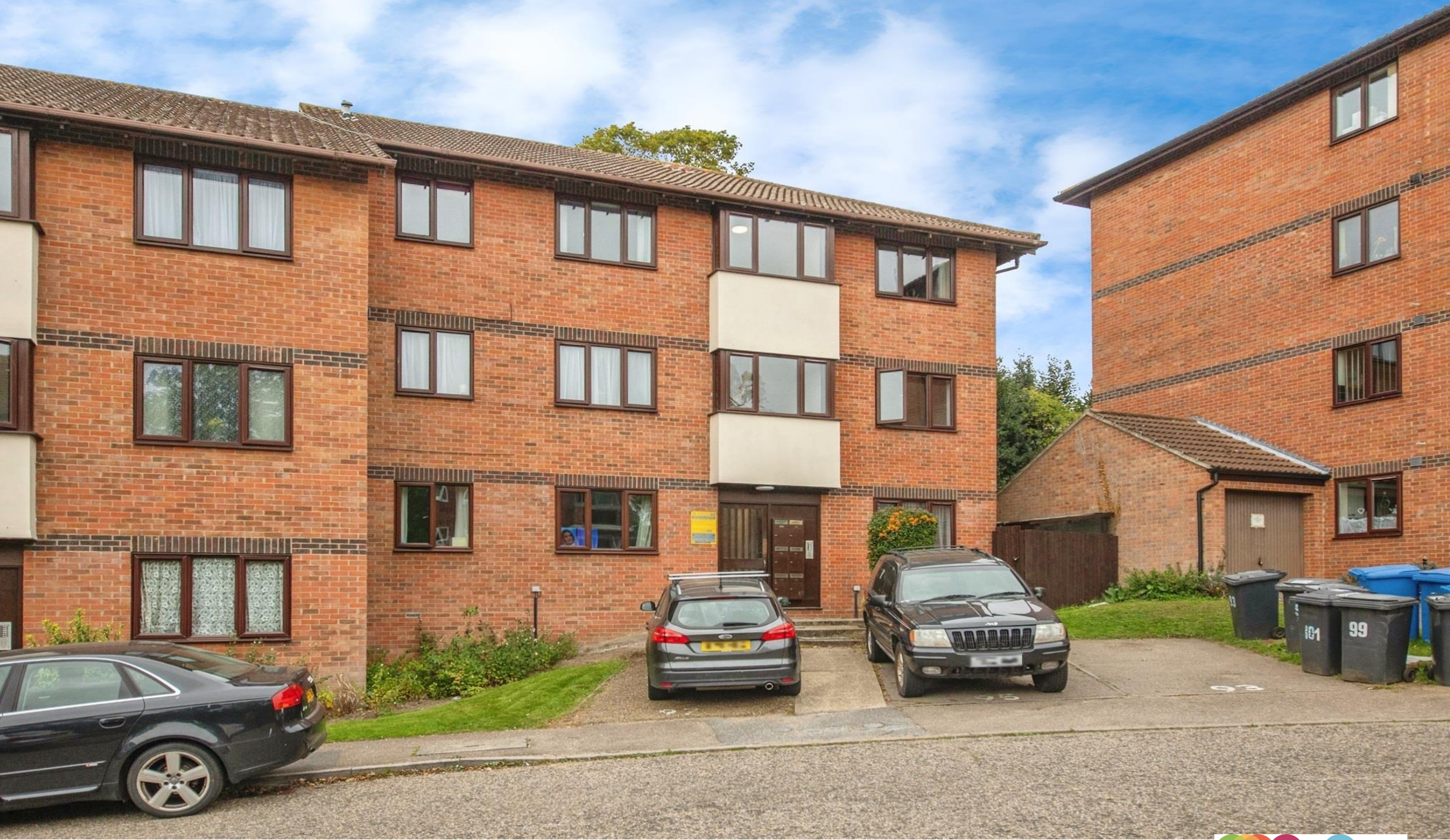
Oakstead Close, Ipswich, IP4 4HW
