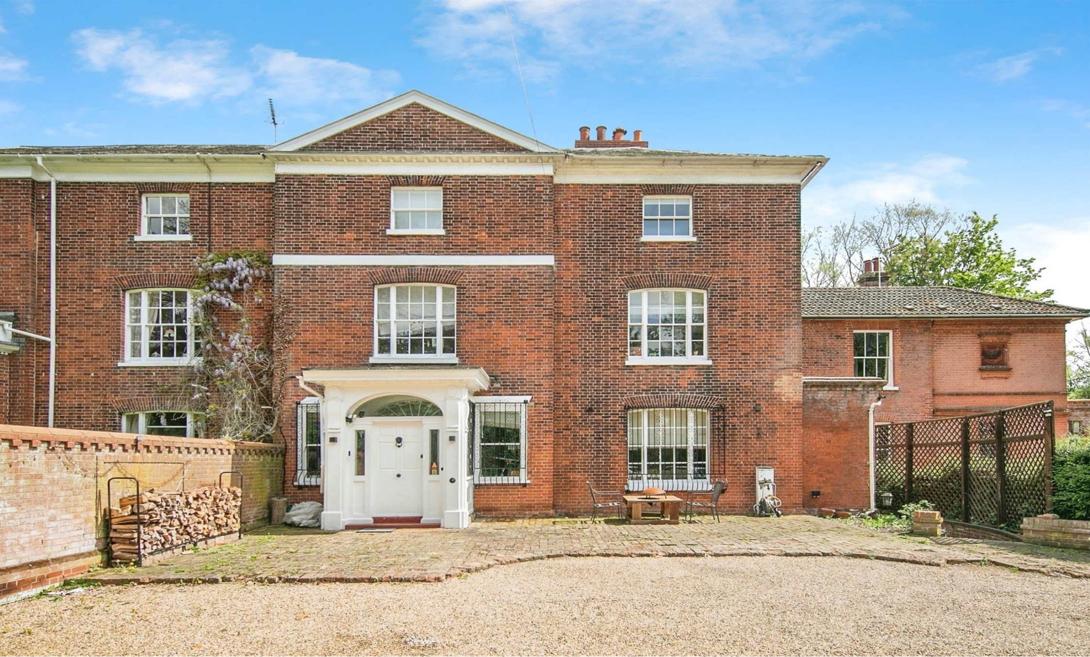
Farah House, Paper Mill Lane, Bramford, IPSWICH, IP8 4BU
