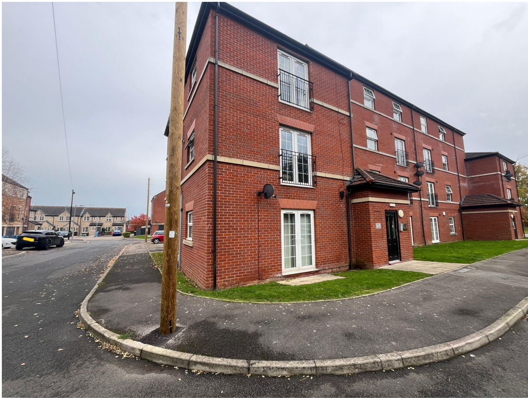
Lambwath Hall Court, Bransholme, Hull, HU7 4WN
