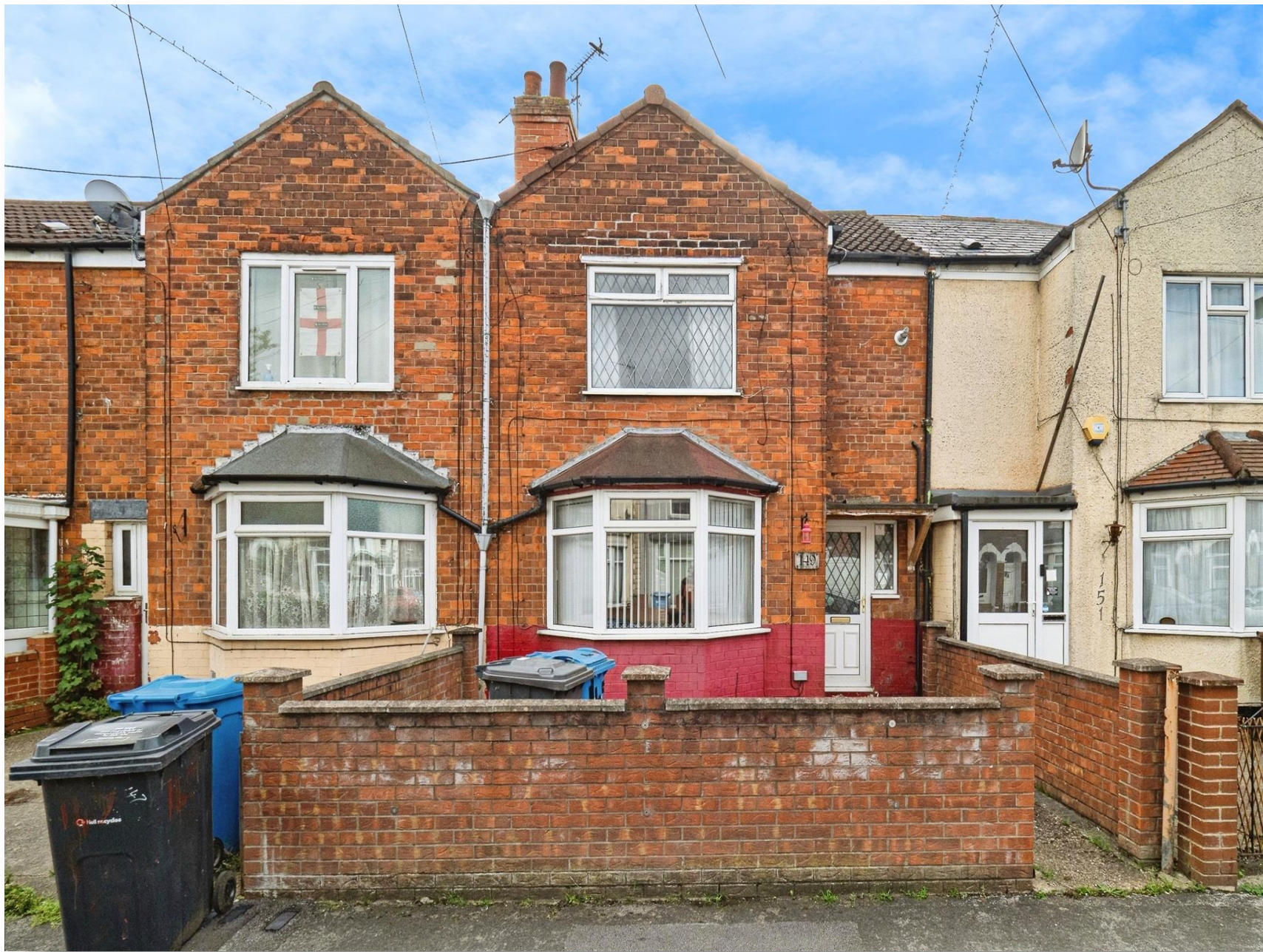
Severn Street, Hull, HU8 8TH
