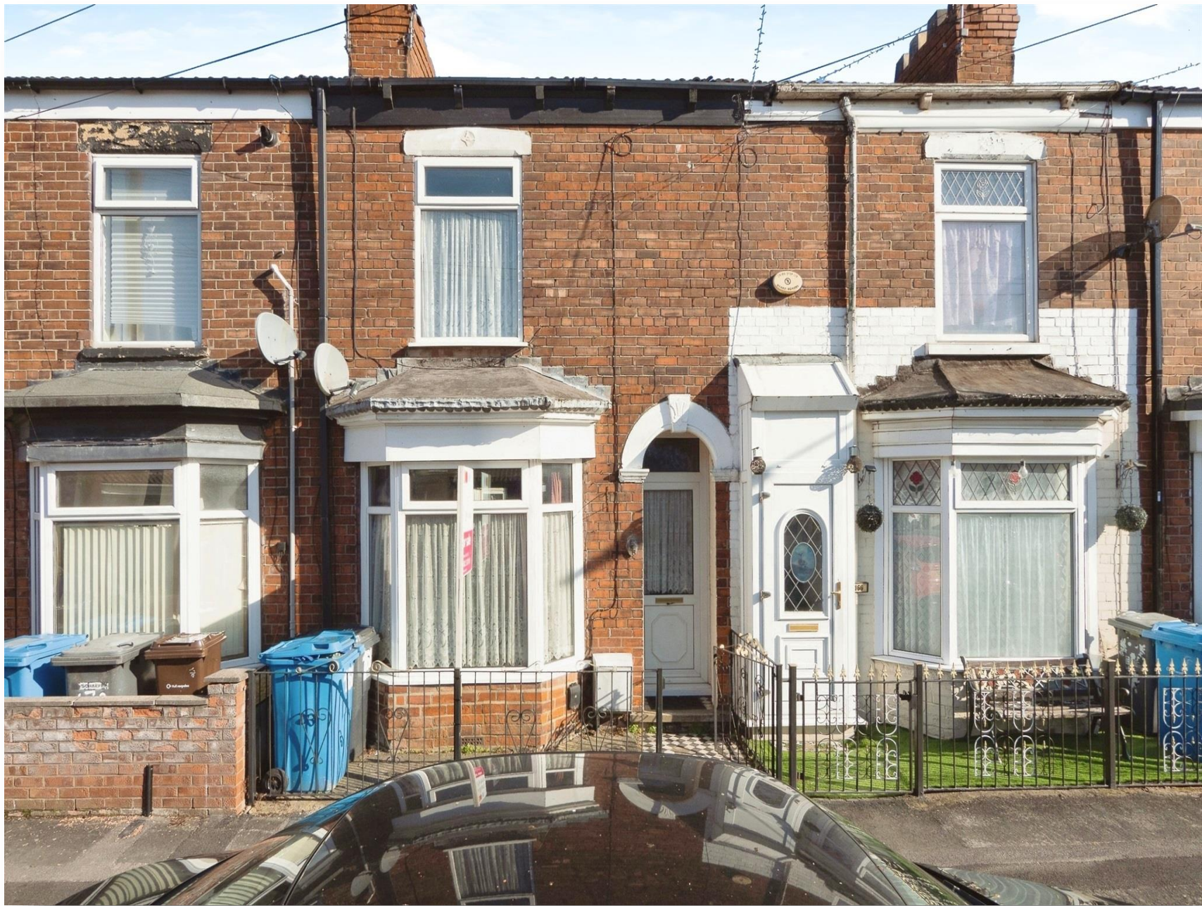
Severn Street, Hull, HU8 8TH
