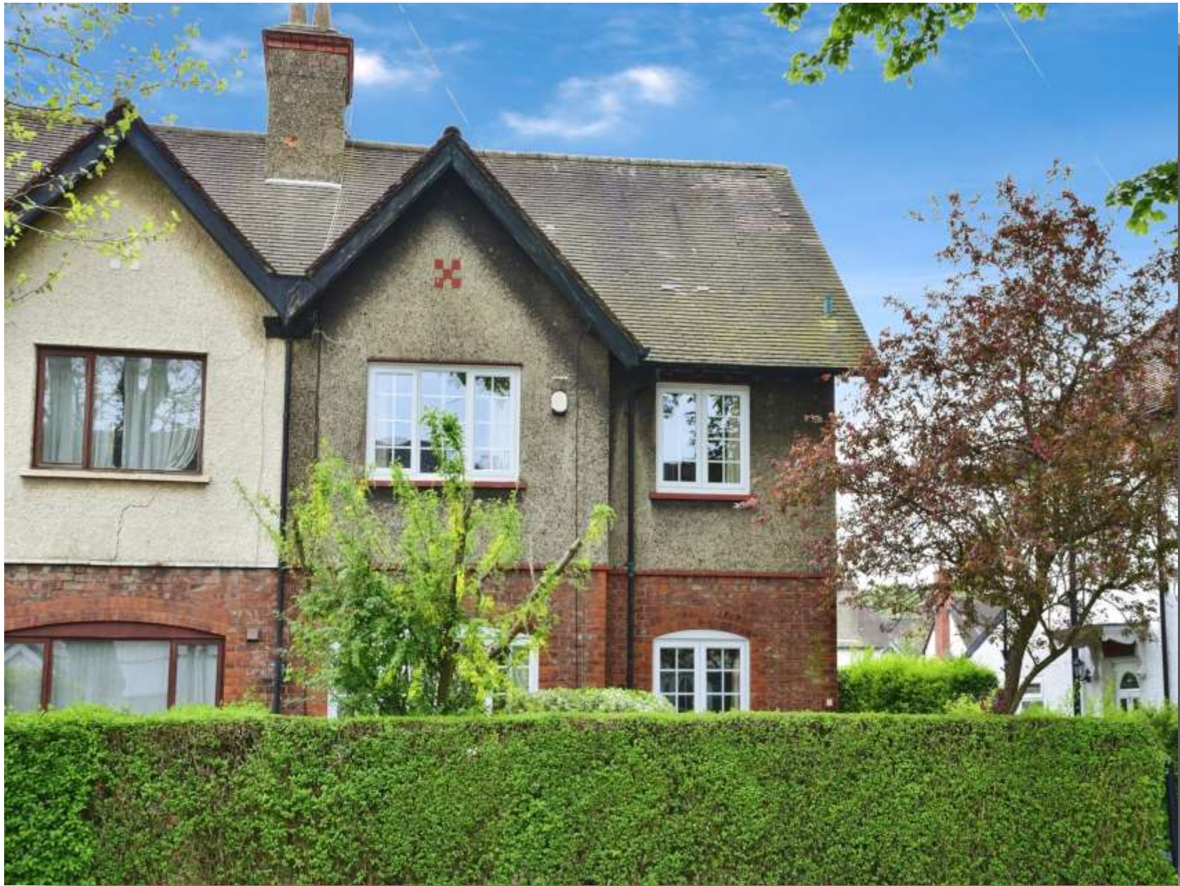
Laburnum Avenue, Garden Village, Hull, HU8 8PH
