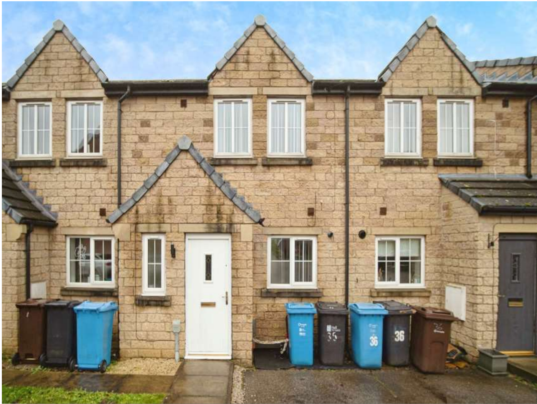
Lambwath Hall Court, Bransholme, Hull, HU7 4WN
