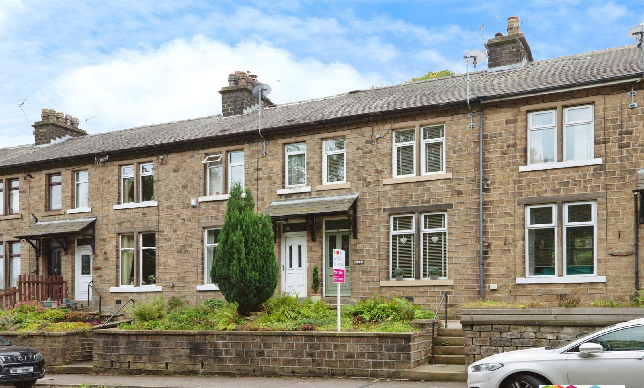
Manchester Road, Linthwaite, Huddersfield HD7 5NE
