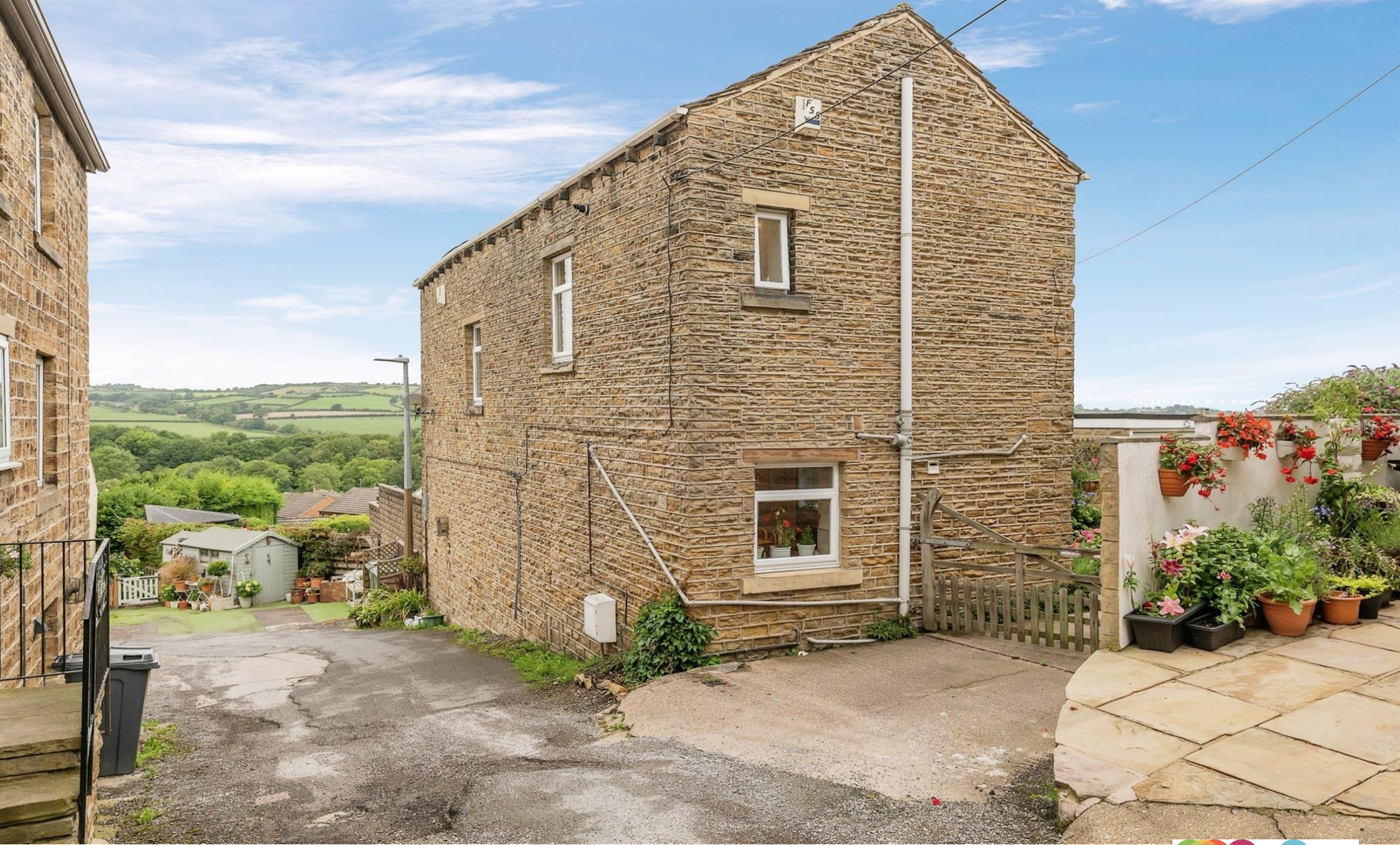
The Ings, Clayton West, Huddersfield HD8 9NJ
