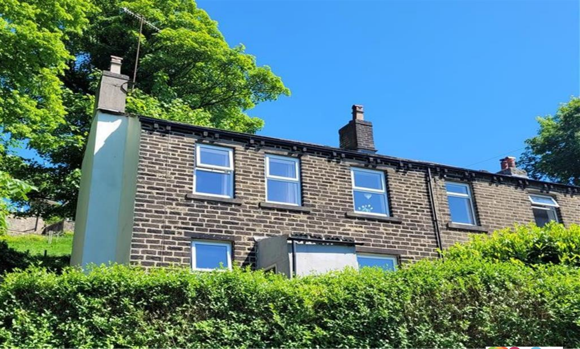
Bank End Cottage, Lea Lane, Netherton, Huddersfield HD4 7DP
