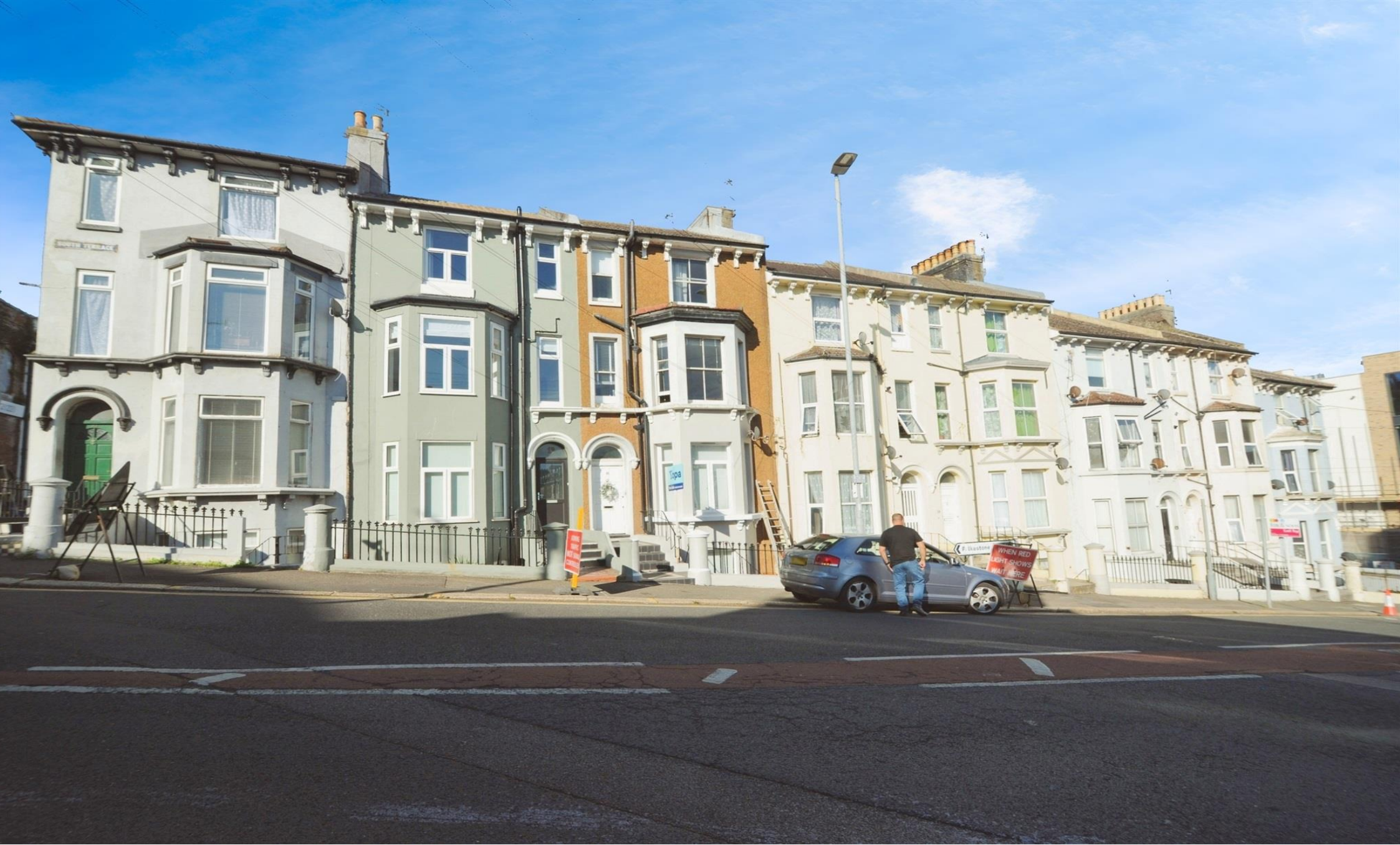
Upper Maisonette South Terrace, Hastings TN34 1SD
